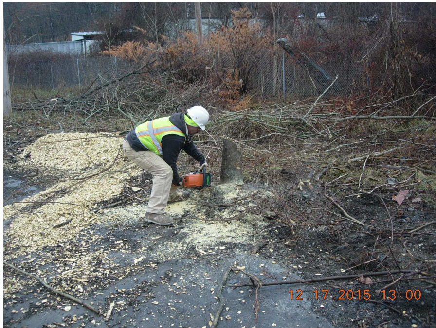
Cutting stump to ground level
