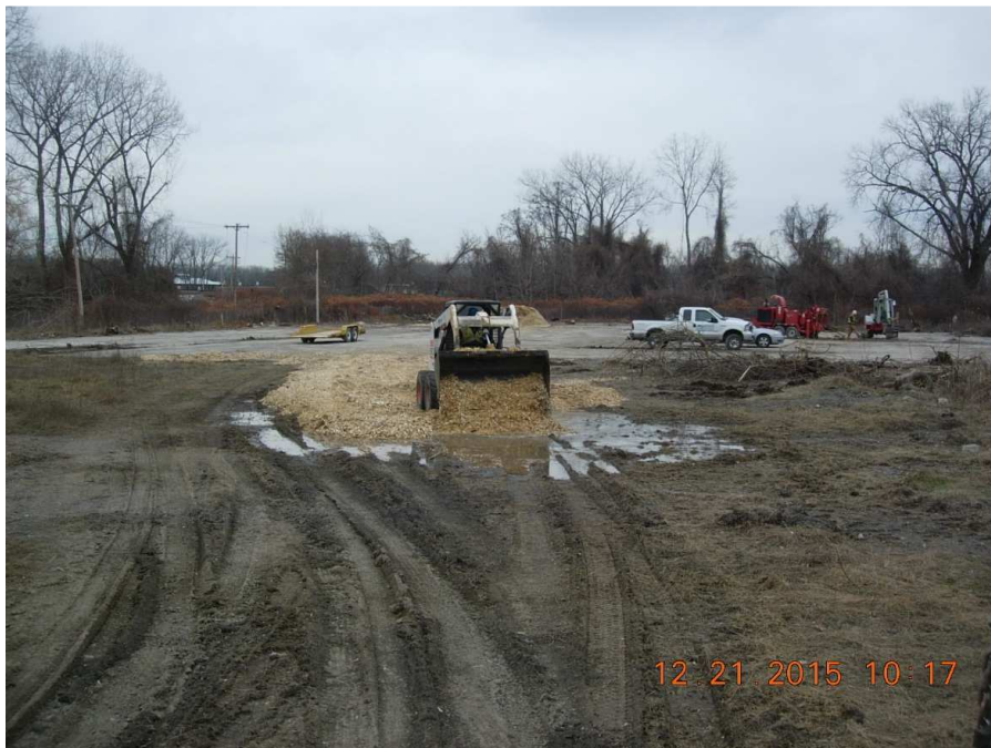
Spreading wood chips on access road
