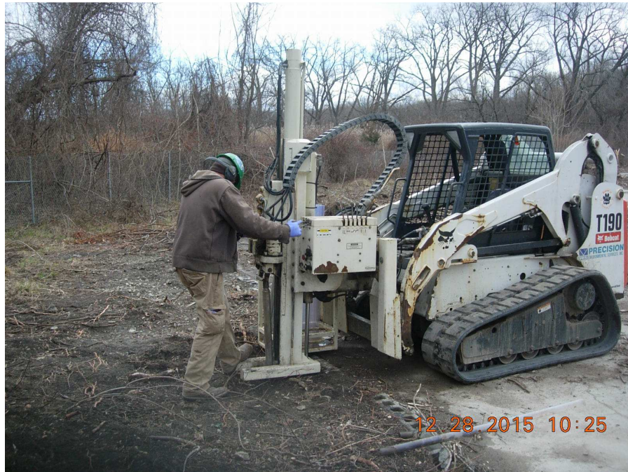
Boring north of concrete slab
