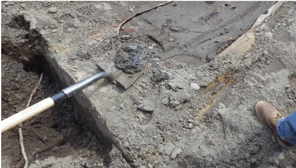
Contaminated soil with oil from UST tank
