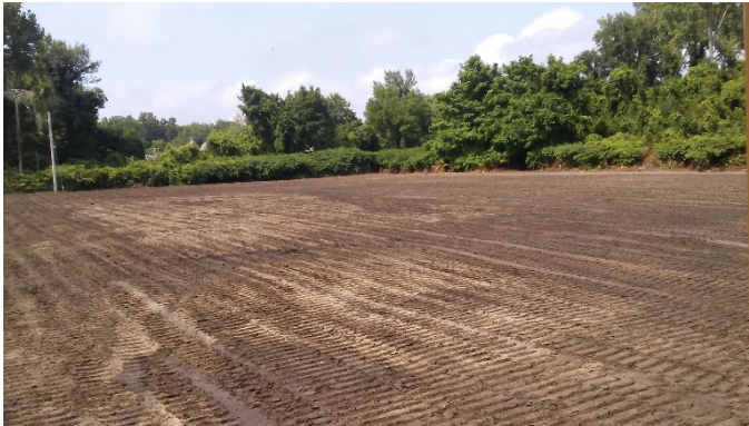
Topsoil applied to rear of site at cut areas
