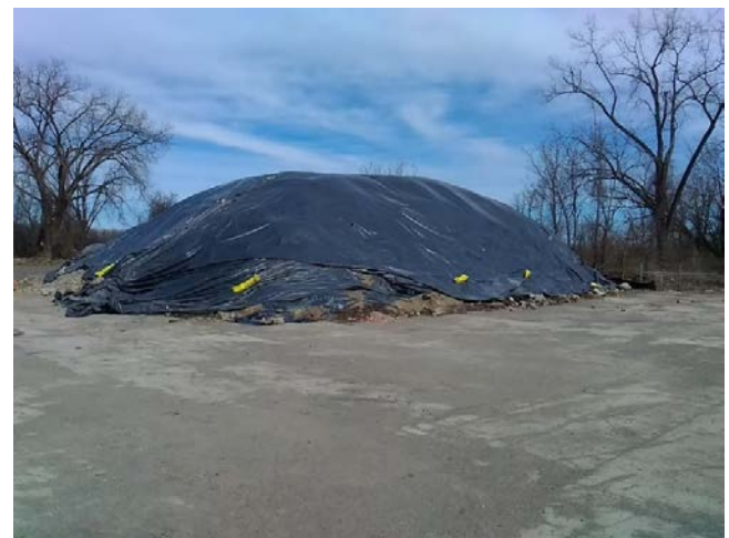
Poly-encapsulated cut soils
