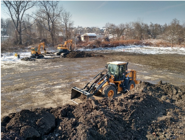
Employing cut and fill methods to remove the top 2-ft of existing soil and apply 1.5-ft of select fill over Demarcation layer and beneath topsoil cover
