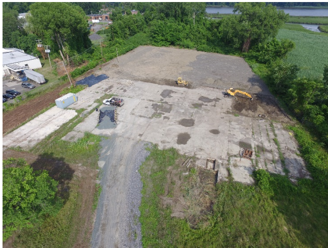
Final cut and select fill application at rear cut area
