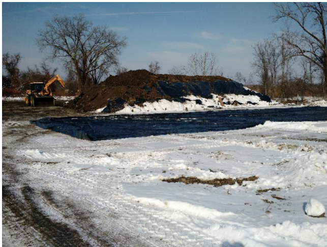
Cut soil staging area
