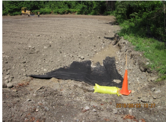
Select fill applied over demarcation layer
