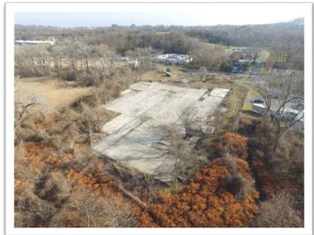
Post demolition aerial view of site
