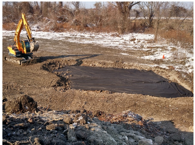
Employing cut and fill methods to remove the top 2-ft of existing soil and apply 1.5-ft of select fill over Demarcation layer and beneath topsoil cover
