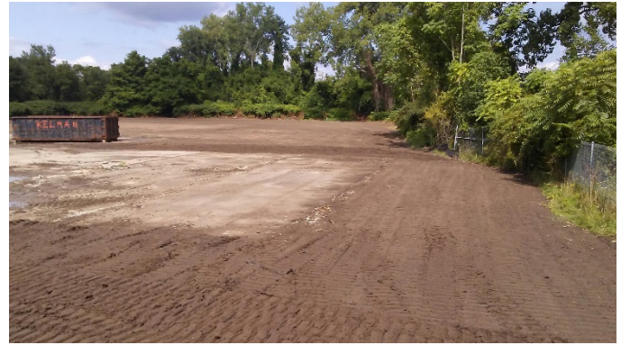
Topsoil applied to north side and front of site
