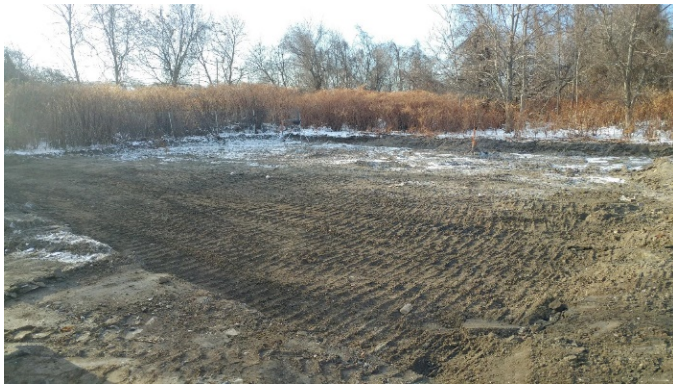
Initial 2-ft cut at SW corner of site
