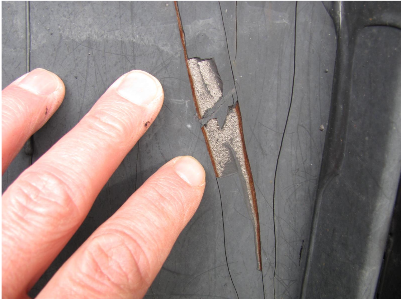
Photo 3 – Typical vertical coating cracks. Note through-crack rust.
