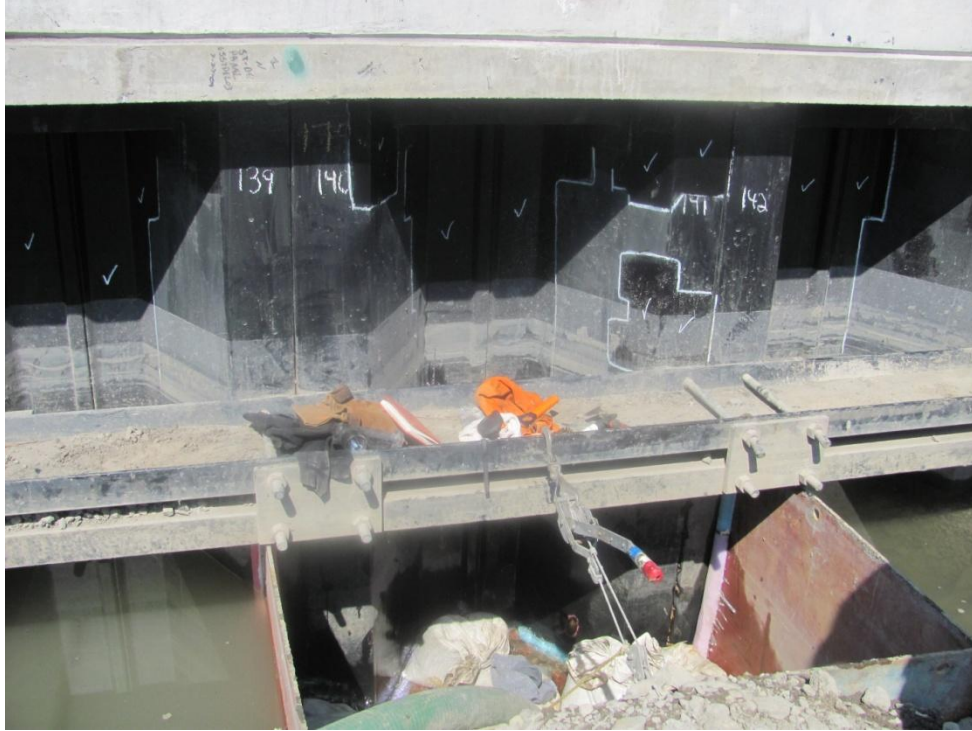
Photo 6 – Overview of 1P175/1P176 excavation area.
