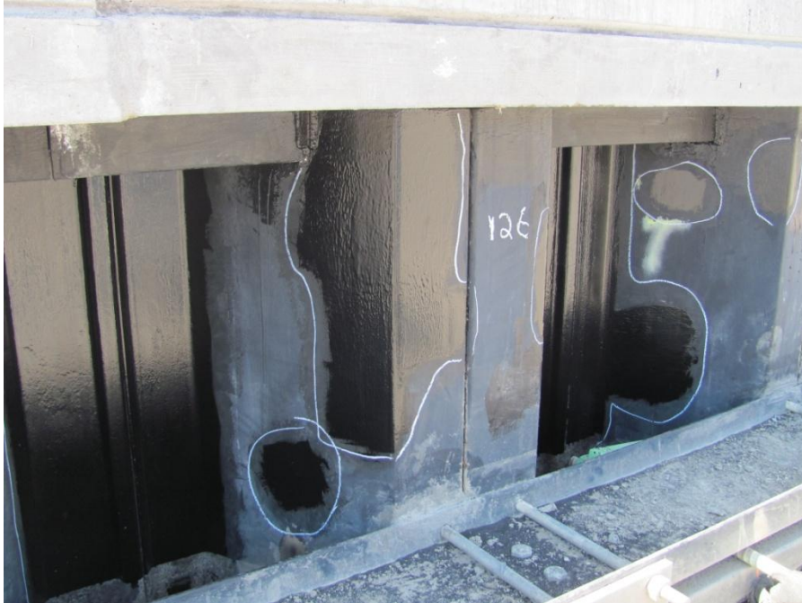
Photo 5 –Overview of Zone 1 repair areas.
