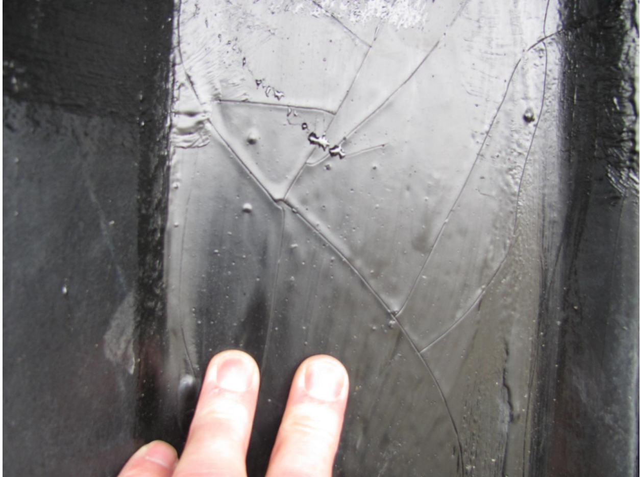
Photo 7 – Overcoating of cracks.
