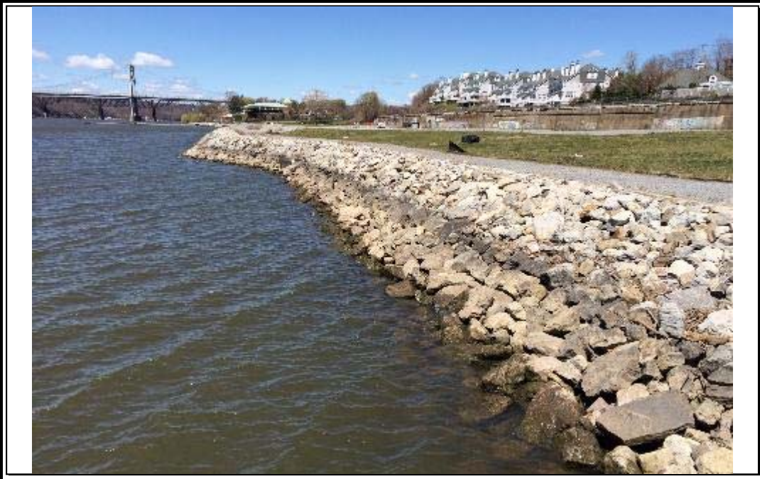
Photo 5 – Looking north; Zone 2 riprap revetment.
