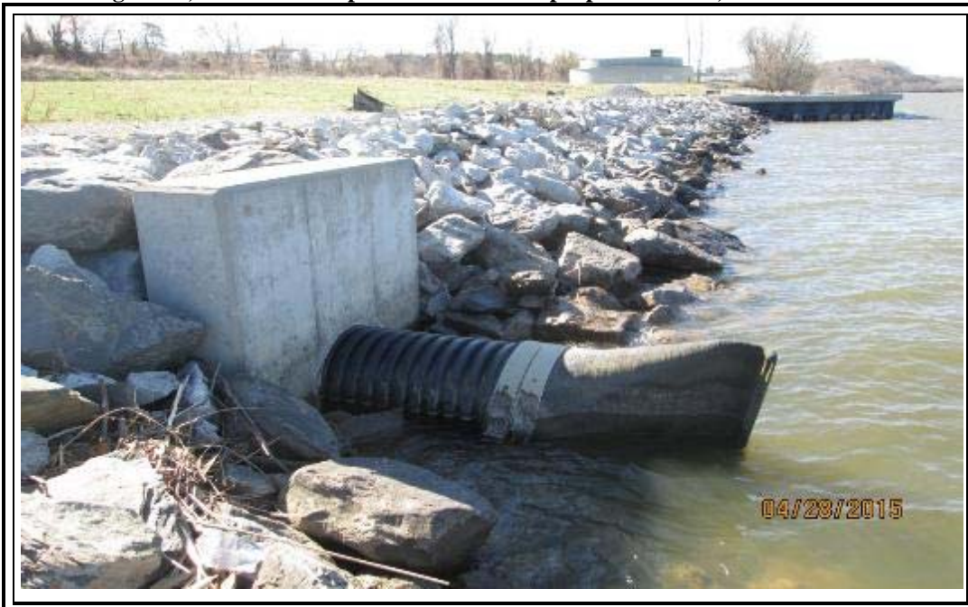
Photo 12 –Looking south, southeast; outfall/ drainage structure within southern portion of Zone 2 riprap revetment.
