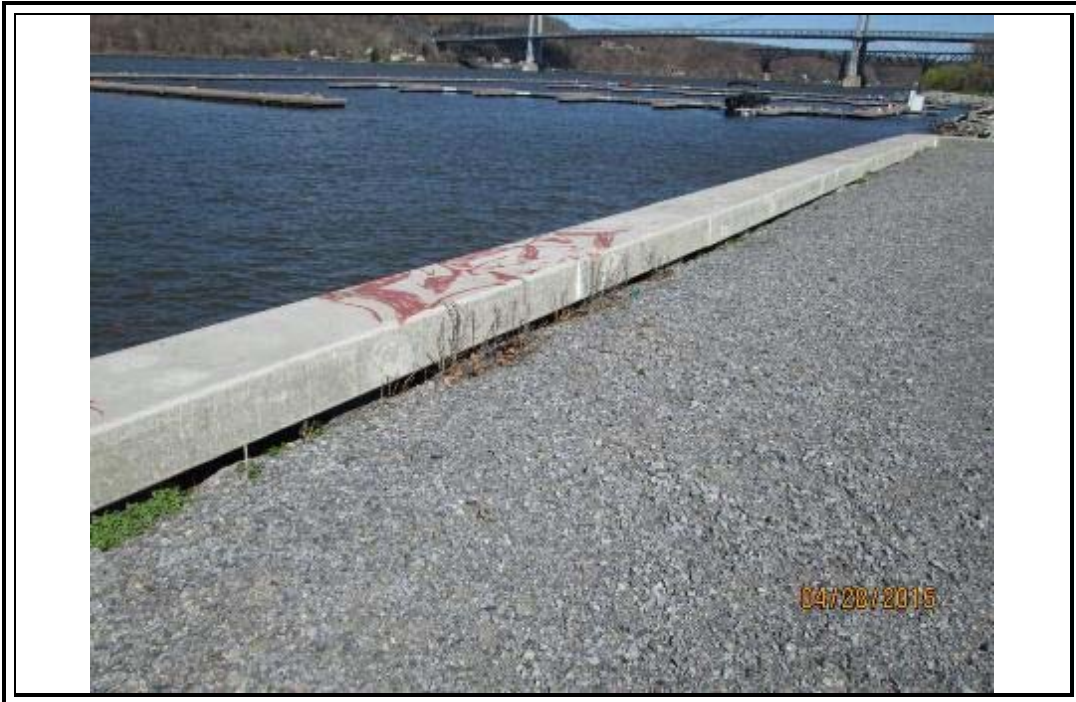
Photo 27 – Looking northwest; northern portion of Zone 3 bulkhead; note settlement of fill behind sheet piles, beneath concrete cap.
