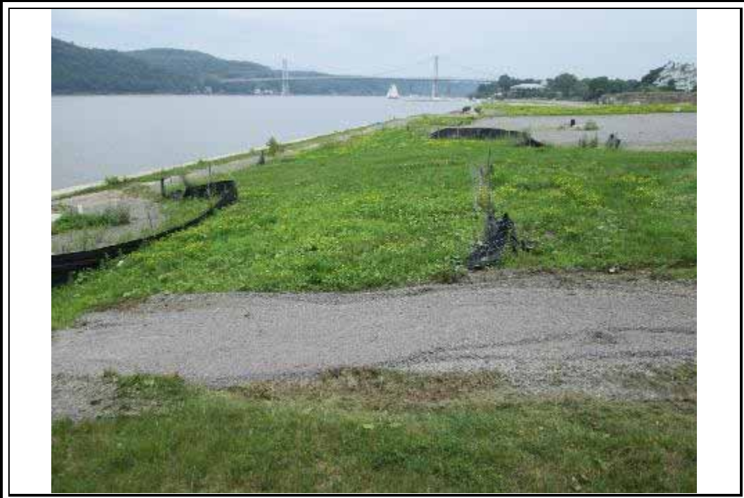
Photo 73 – Repaired scour at the southern end of Zone 1. (Refer to photo 21)
