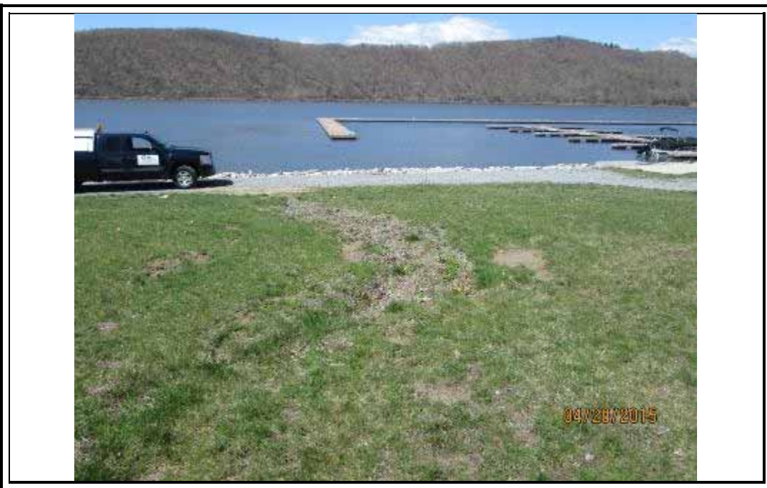
Photo 28 – Looking west; scour near southern end of Zone 4.
