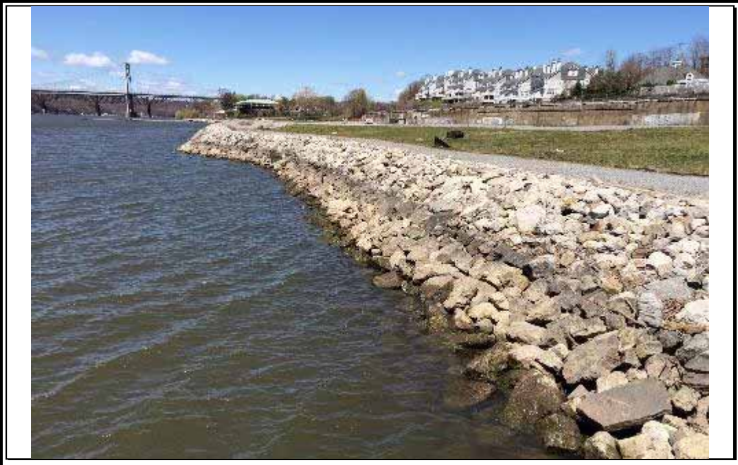
Photo 5 – Looking north; Zone 2 riprap revetment.
