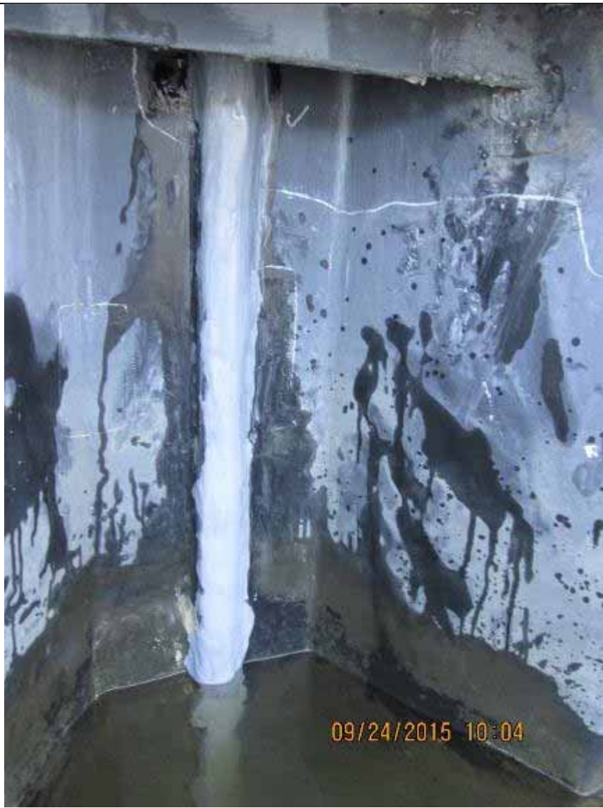
Photo 75 – Repaired sheet pile interlock (Zone 3 Bulkhead) on 9-24-15.
