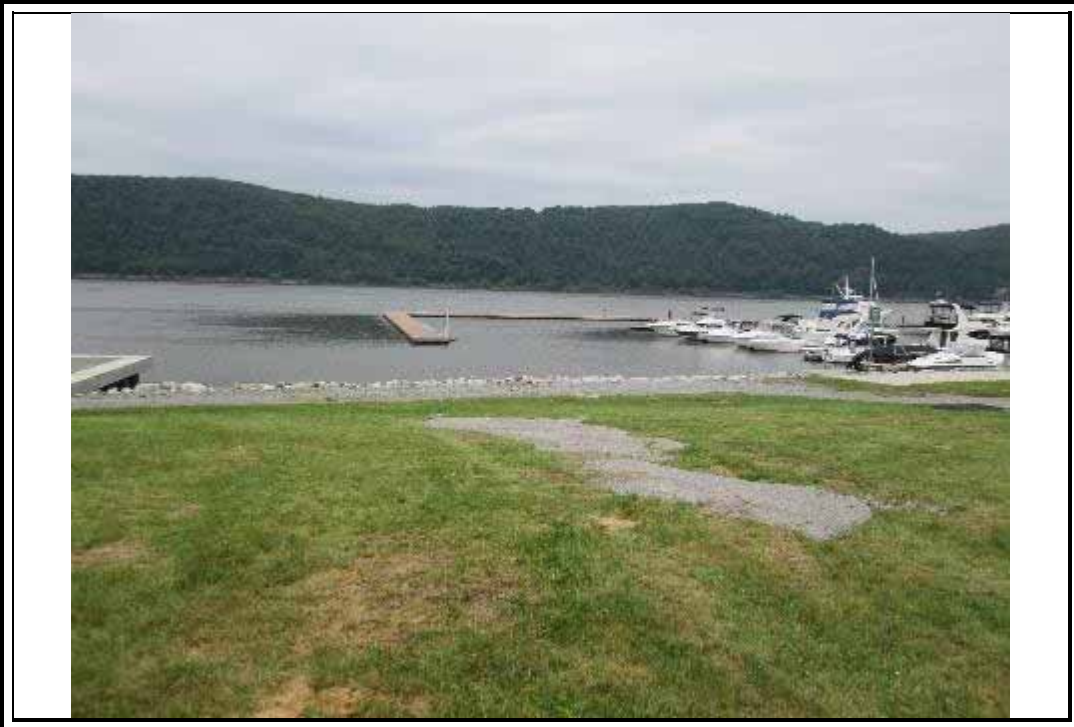
Photo 71 – Repaired scour at the southern end of Zone 4. (Refer to photo 28)
