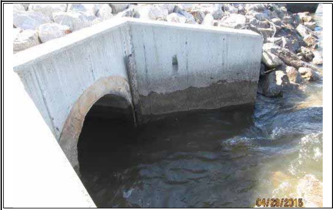
Photo 9 – Looking southeast; outfall/ drainage structure within Zone 2 riprap revetment .
