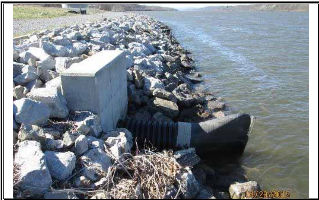
Photo 10 - Looking south; outfall/ drainage structure within Zone 2 riprap revetment.
