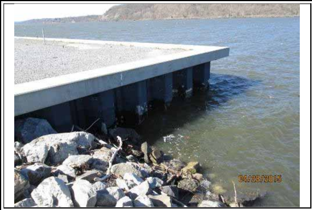
Photo 13 – Looking southwest; northern end of Zone 1 bulkhead.
