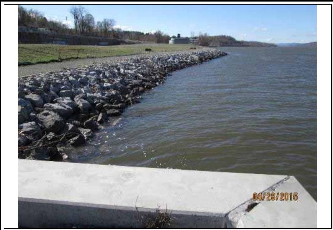
Photo 7 – Looking south; Zone 2 riprap revetment from southern end of Zone 3 bulkhead.
