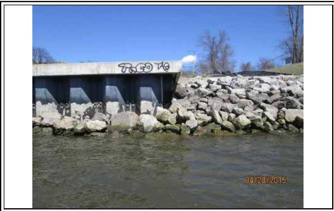
Photo 47 – South end of Zone 1 bulkhead.
