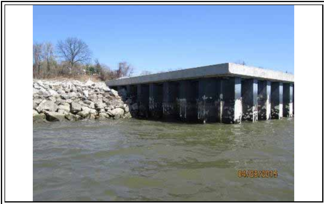
Photo 29 –North end of Zone 1 bulkhead.
