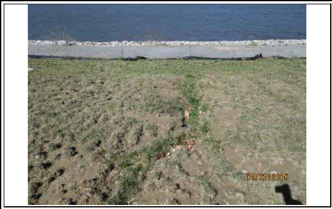
Photo 25 – Looking west; scour at north end of Zone 2.
