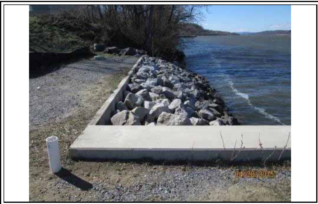
Photo 14 – Looking south; southern end of Zone 1 bulkhead.
