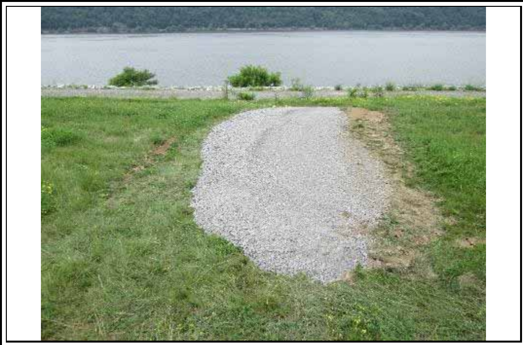
Photo 72 – Repaired scour at the north end of Zone 2. (Refer to photo 25)
