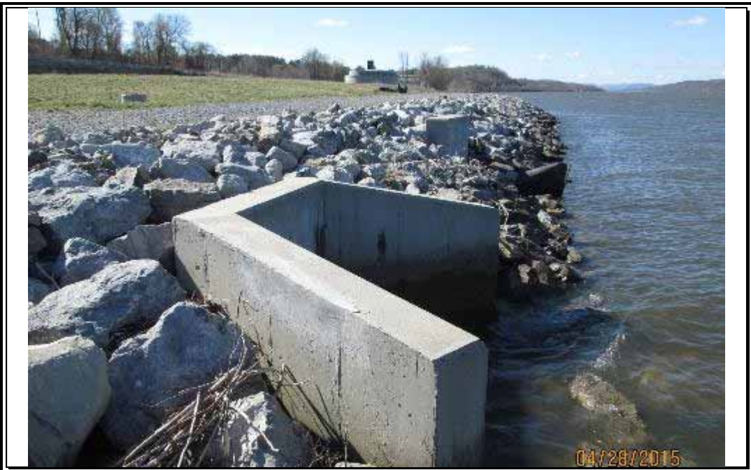
Photo 8 – Looking south; outfall/ drainage structures within Zone 2 riprap revetment.
