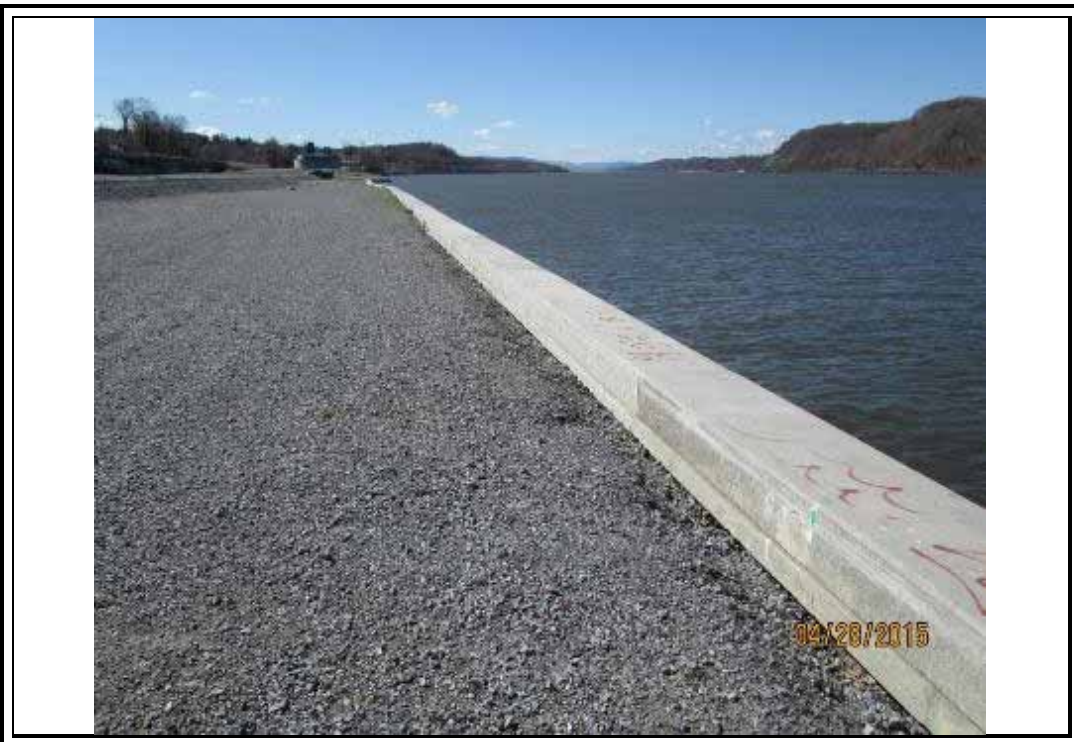
Photo 26 – Looking south; area behind Zone 3 bulkhead.
