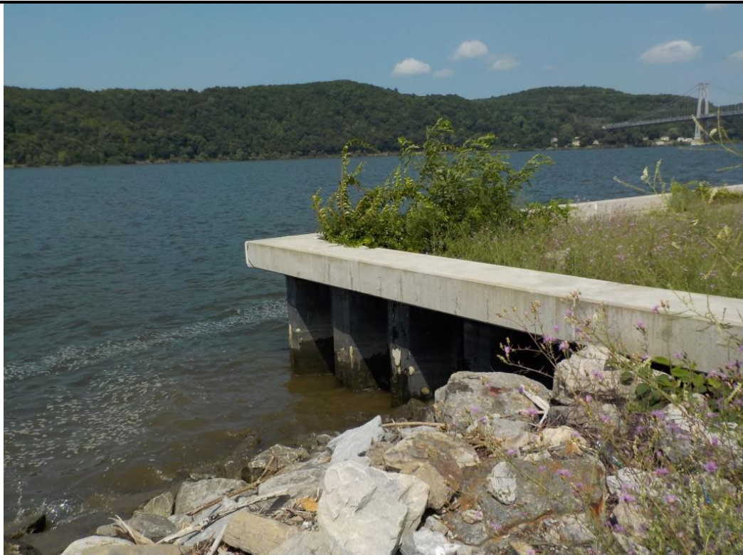
Photograph 8. Minor spalling on bulkhead caps.
