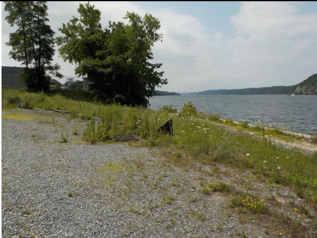
Photograph 7. Fallen silt fence on the south end of the site.
