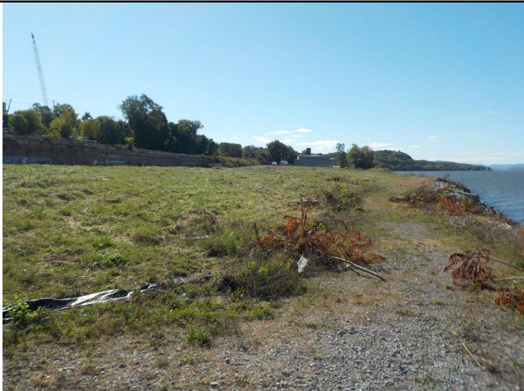
Photograph 8. Fallen silt fence on the northern end of the site.
