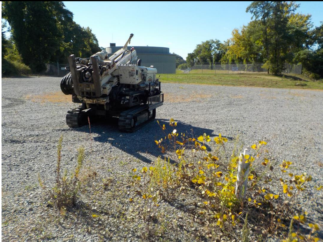
Photograph 9. Drill rig used to re-install replacement monitoring wells MW-4R and MW-7R.
