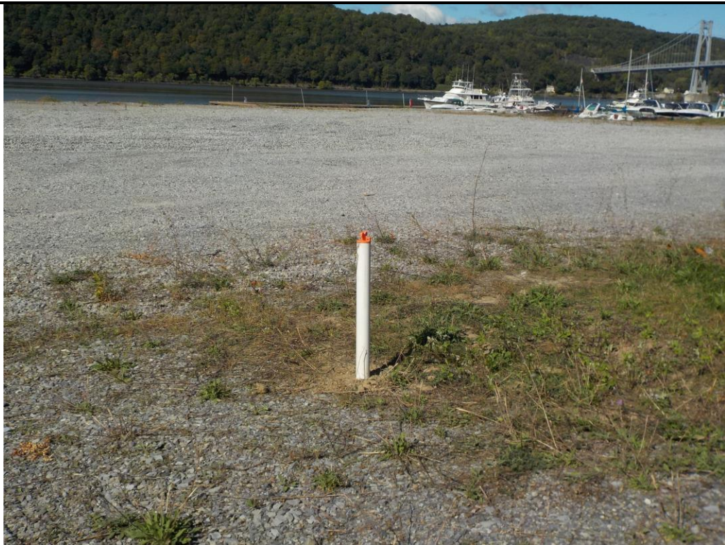
Photograph 2. Re-installation of MW-7 on the DeLaval Property.
