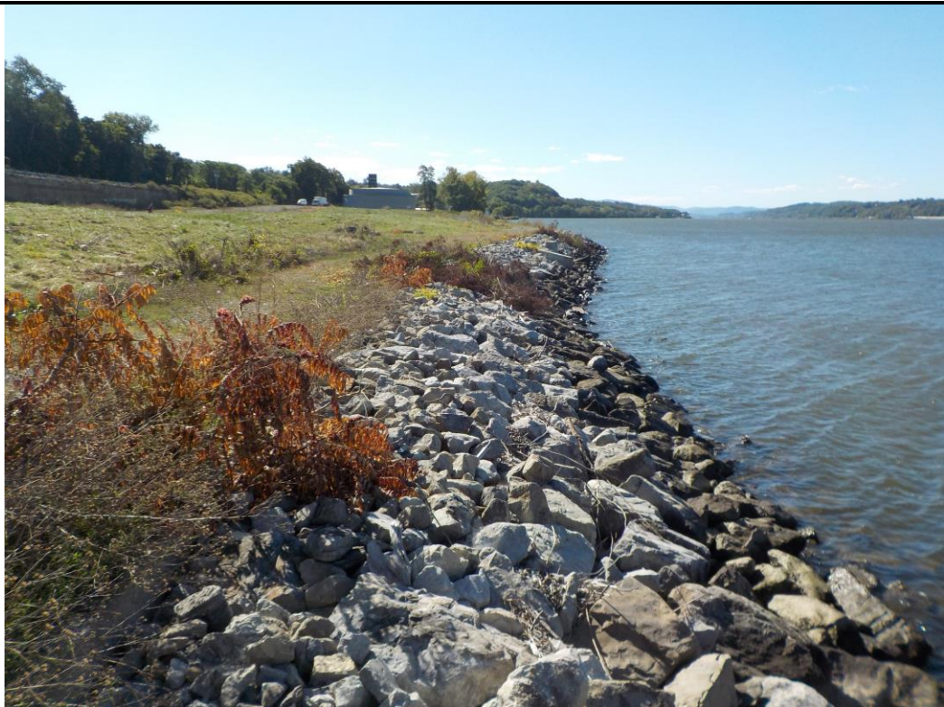
Photograph 10. Stabilization using rip-rap along the Hudson River, looking south.
