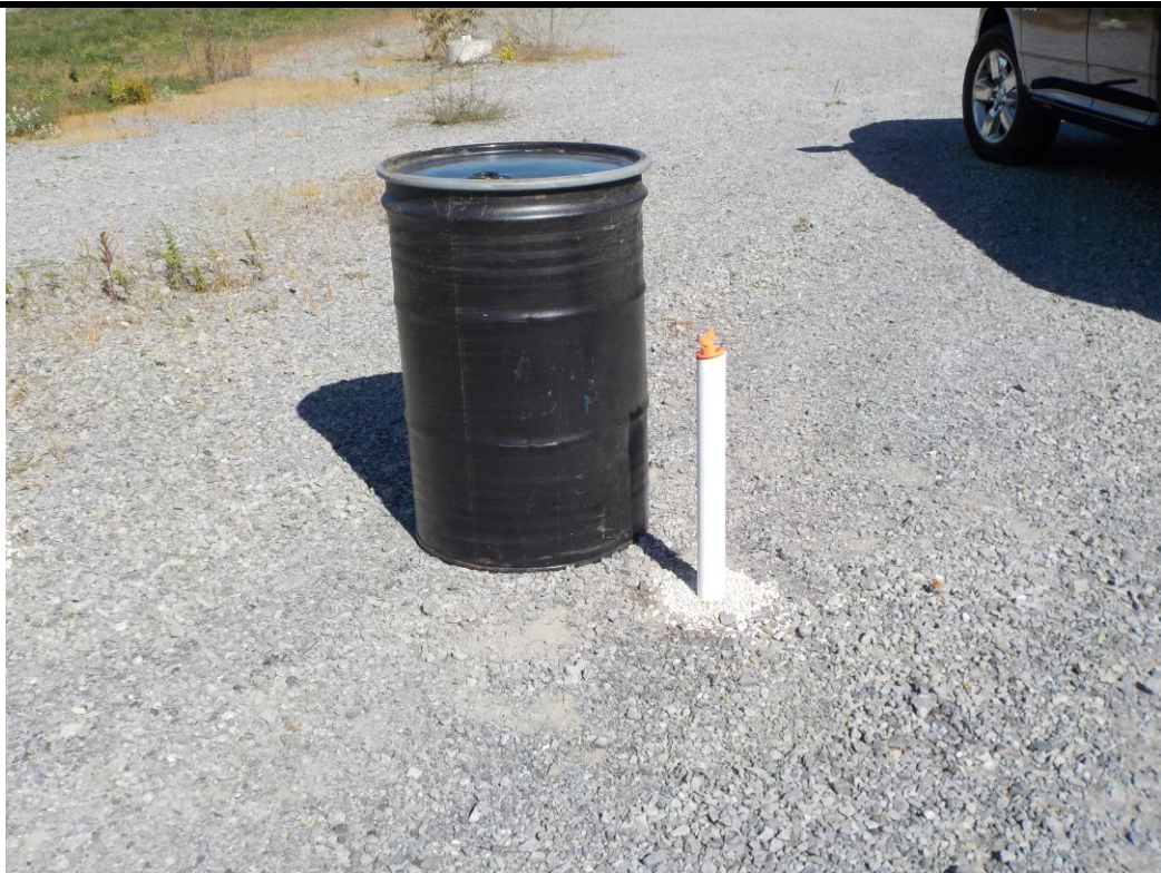
Photograph 1. Re-installation of MW-4 on the DeLaval Property.
