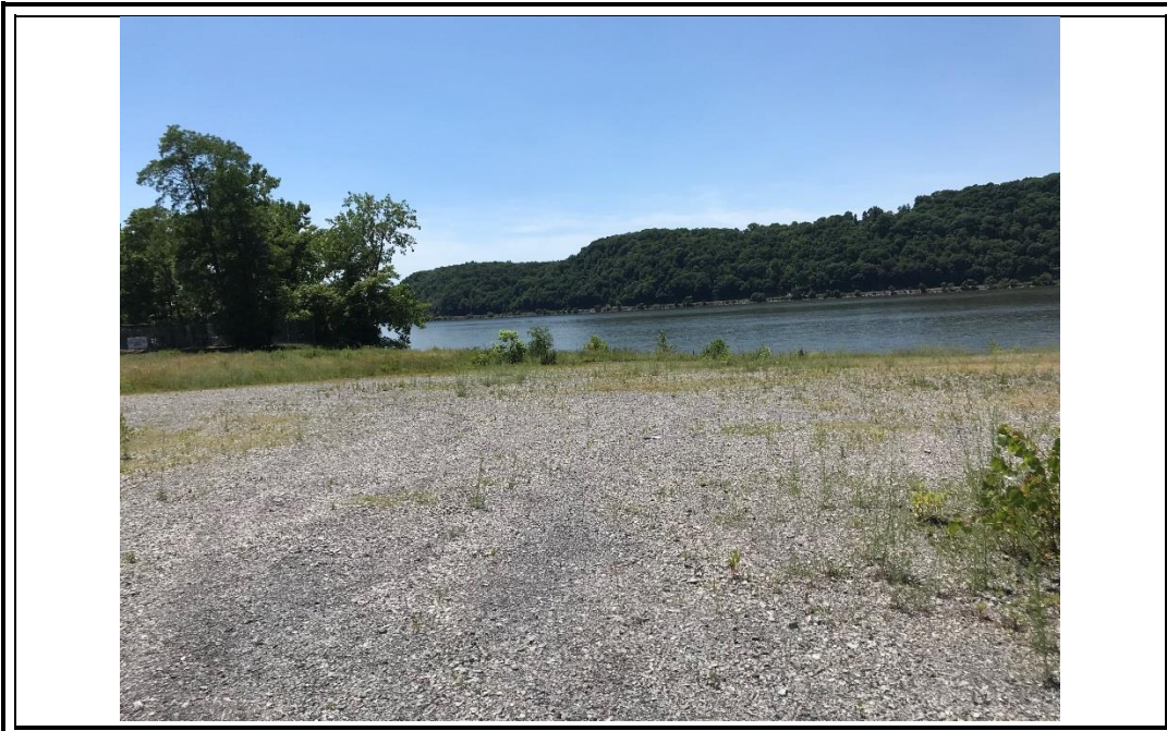
Photograph 12. Looking southeast an example of the run of crush cover system.
