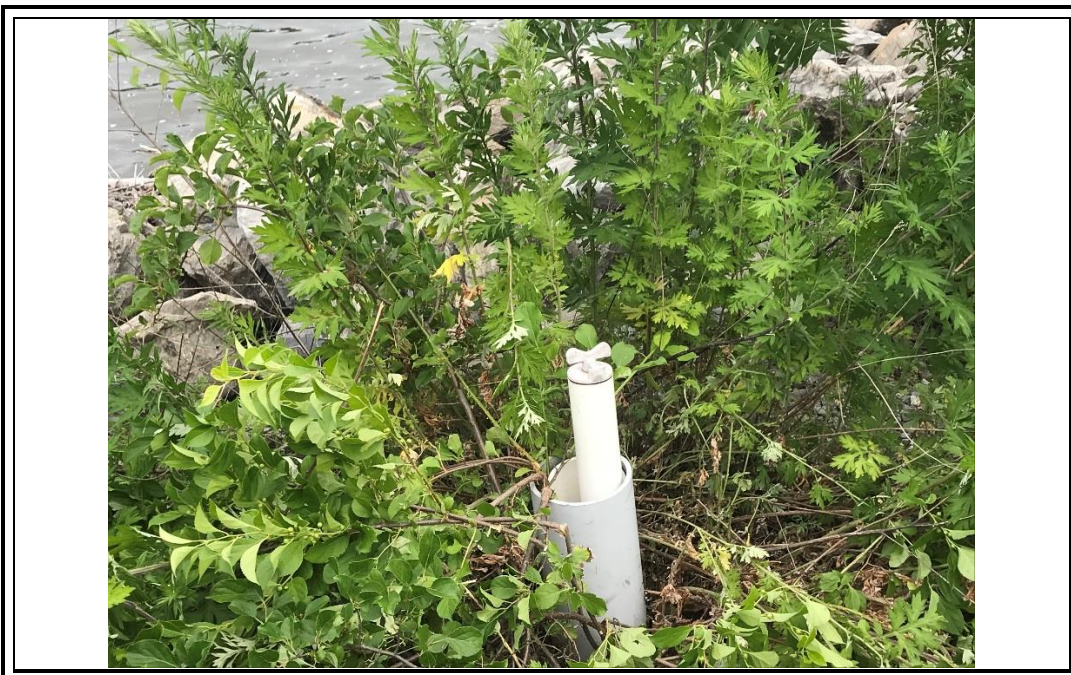
Photograph 18. Example of vegetation ground in and around the PVC casing around the monitoring well.
