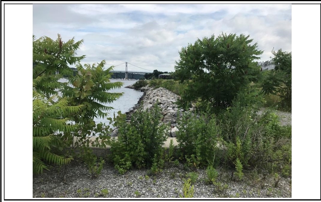
Photograph 17. Rip-rap revetment system on the shore of the river, looking north.
