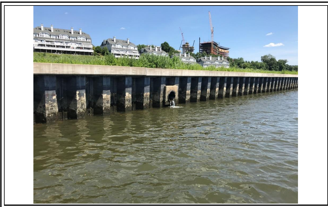
Photograph 14. Zone 3 Bulkhead and the concrete headwall at outfall.
