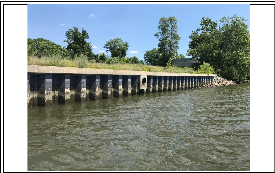
Photograph 16. Zone 1 Bulkhead and concrete headwall at outfall.
