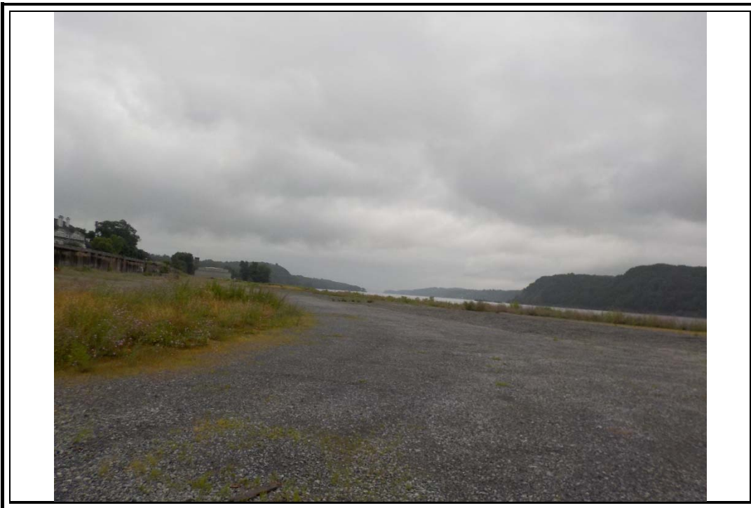
Photograph 4. Stone drive near bulkheads.
