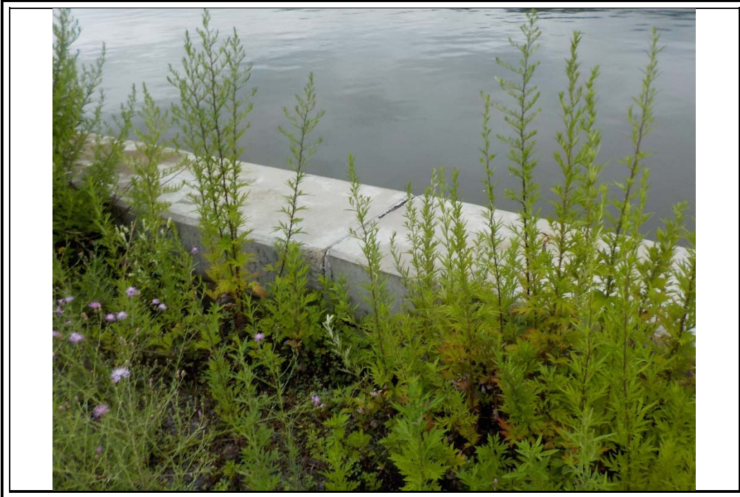
Photograph 5. Spreading between bulkhead caps.
