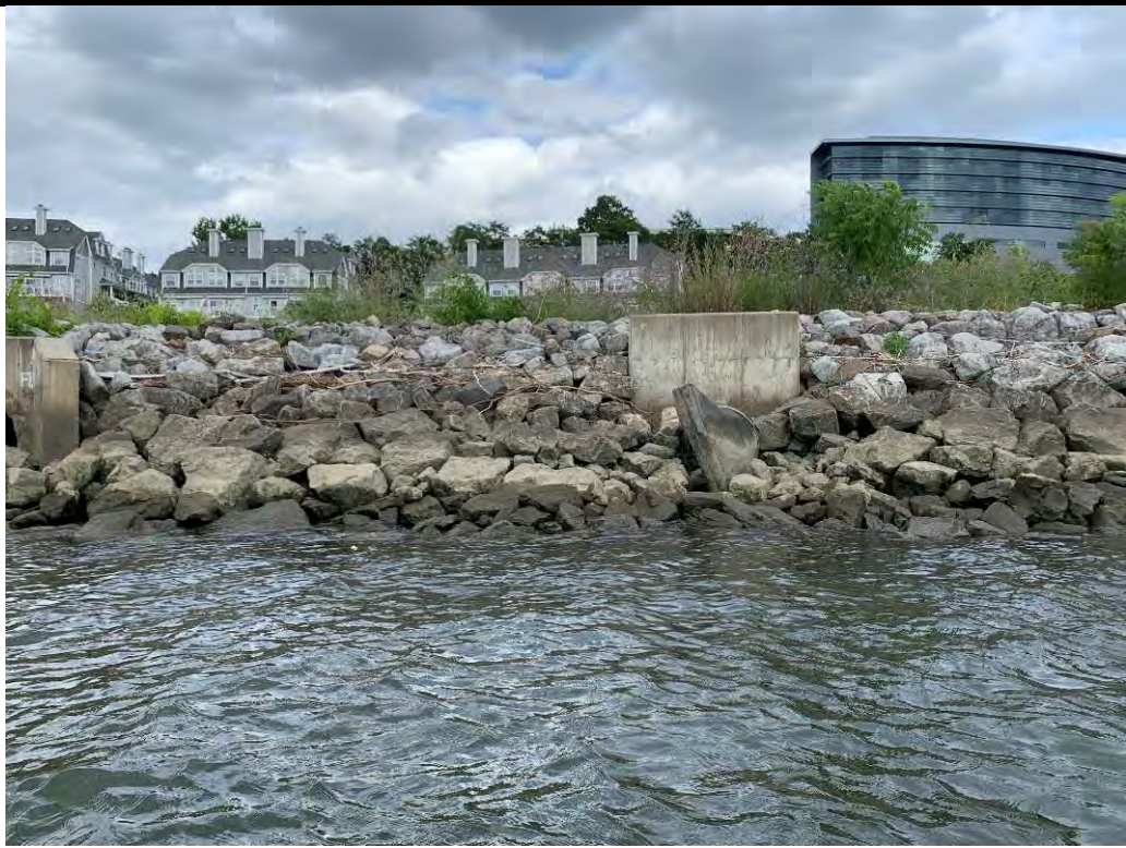
Photograph 9. Riprap stone along Zone 2.
