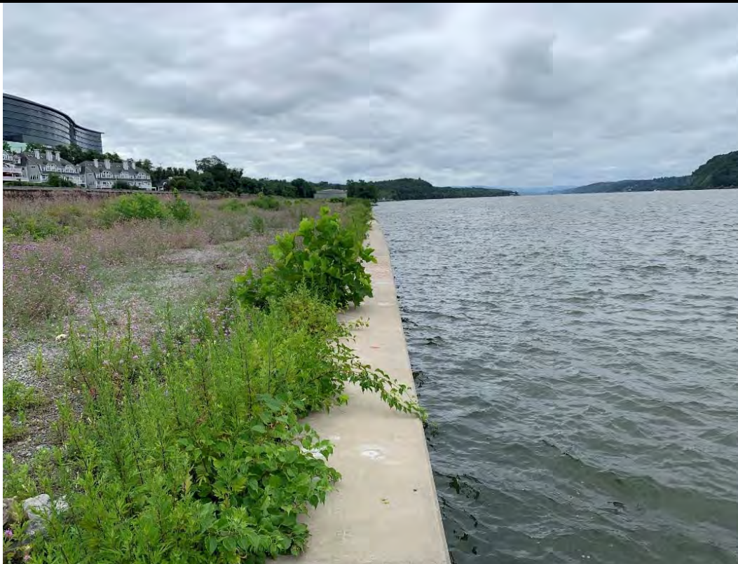
Photograph 4. Looking south along the bulkhead.
