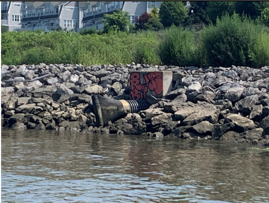
Photograph 8. Riprap stone along Zone 2.
