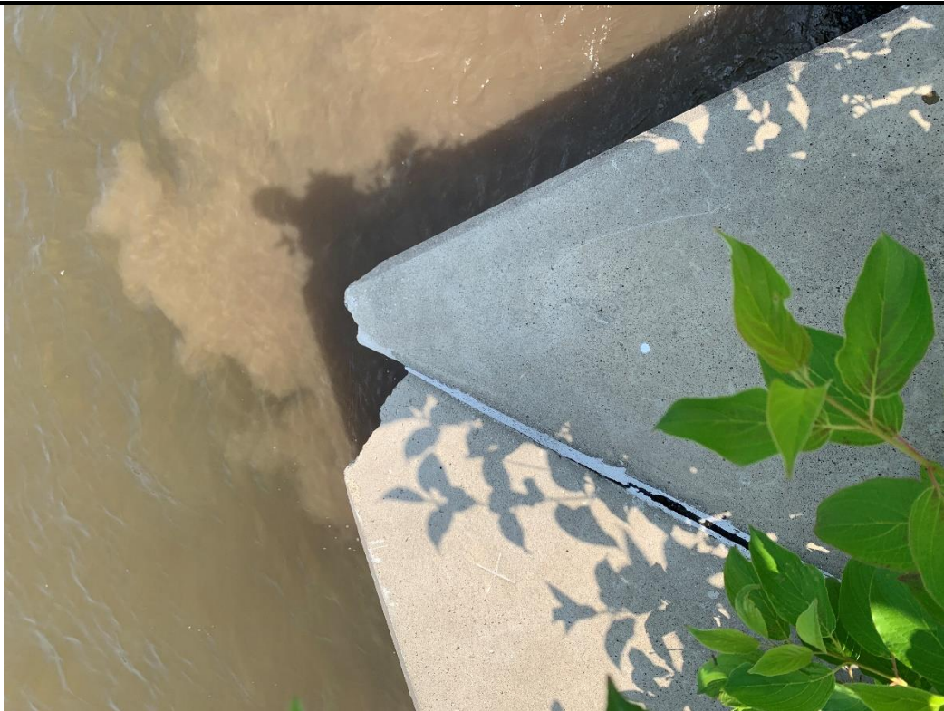
Photograph 10. Corner of concrete cap on bulkhead on the far north end of the subject site.
