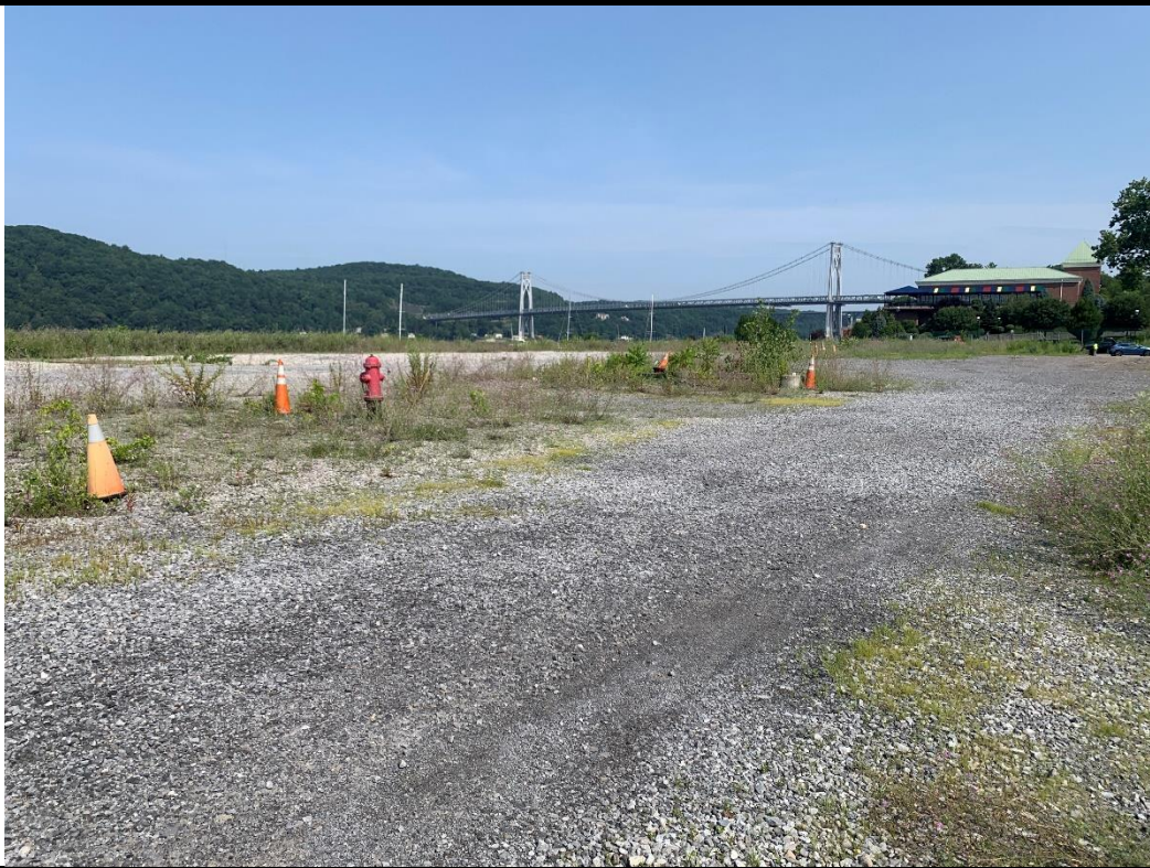
Photograph 1. Site overview facing north.
