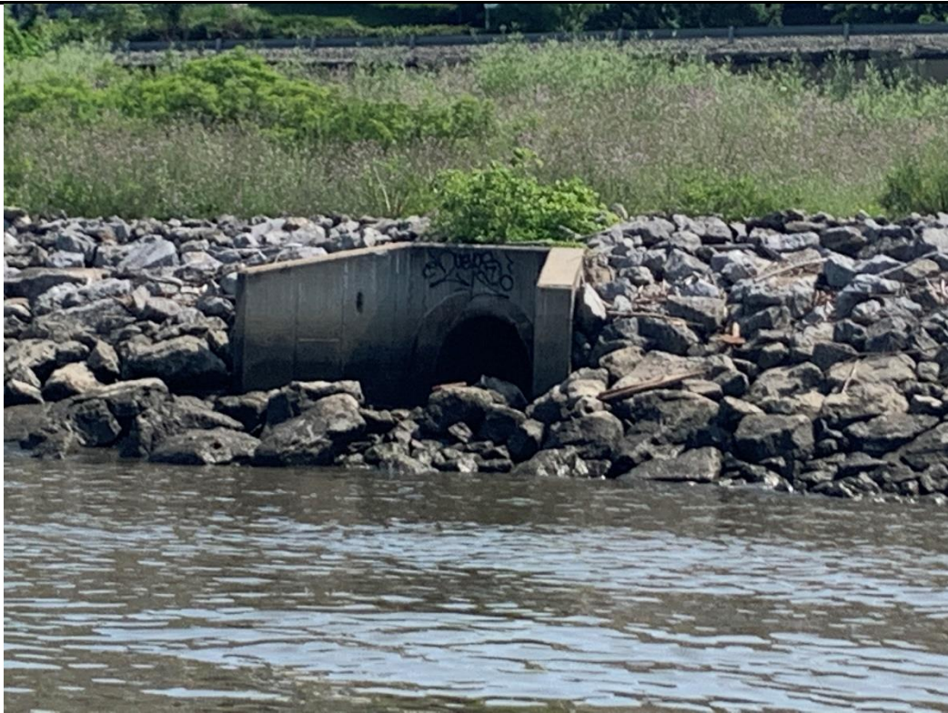
Photograph 12. Culvert cleared with no visible debris.
