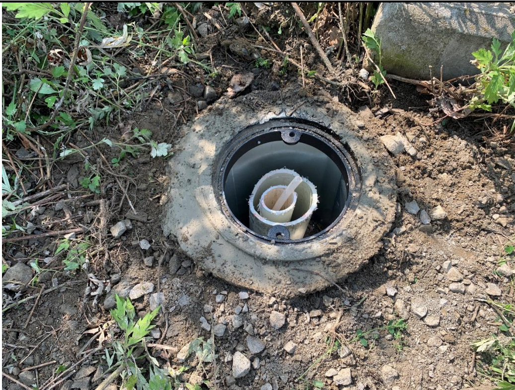
Photograph 14. Permanent flush mount well casing installed at one out of nine monitoring wells.
