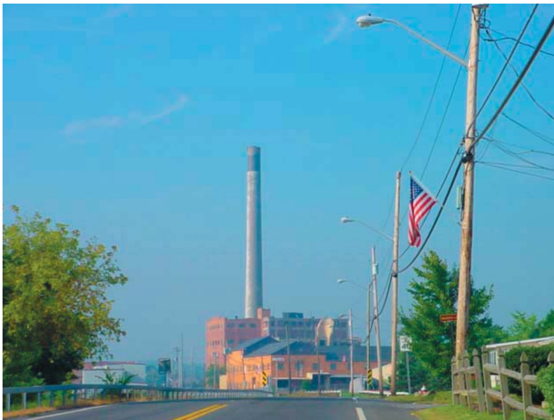
Photo 2 A 2002 photograph of the boiler house and Polyset Company facing south along U.S. Route 4.
