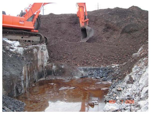
Photo 17 Excavation of contaminated soil.
