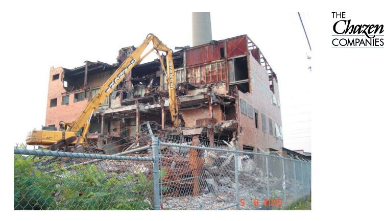
Photo 16 2005 - Demolition of the boiler house and recycling of lead-painted steel.
