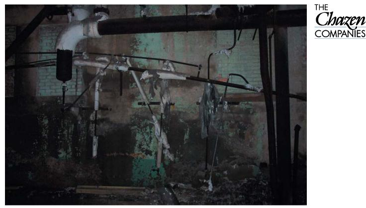
Photo 14 Suspected asbestos containing material on indoor piping.
