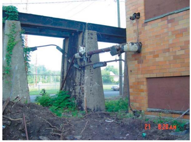
Photo 12 Suspected asbestos containing material insulating outdoor piping.
