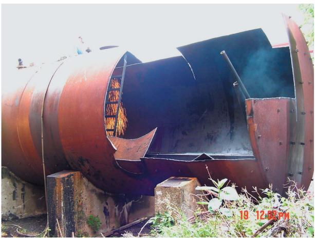
Photo 4 2004 - Cristo Demolition cutting and recycling the 16,000-gallon AST.
