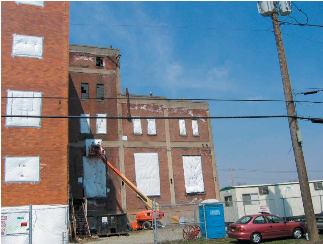
Photo 1 Preparations for asbestos abatement.
