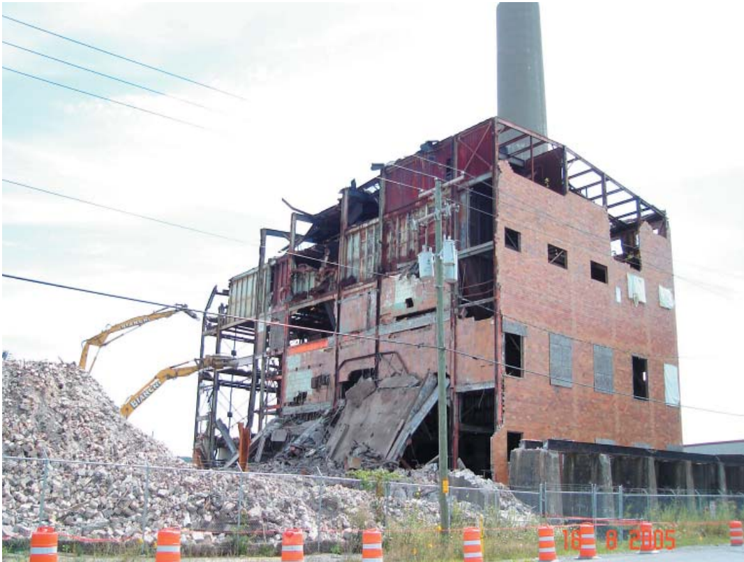
Photo 15 Demolition of south boiler house.
