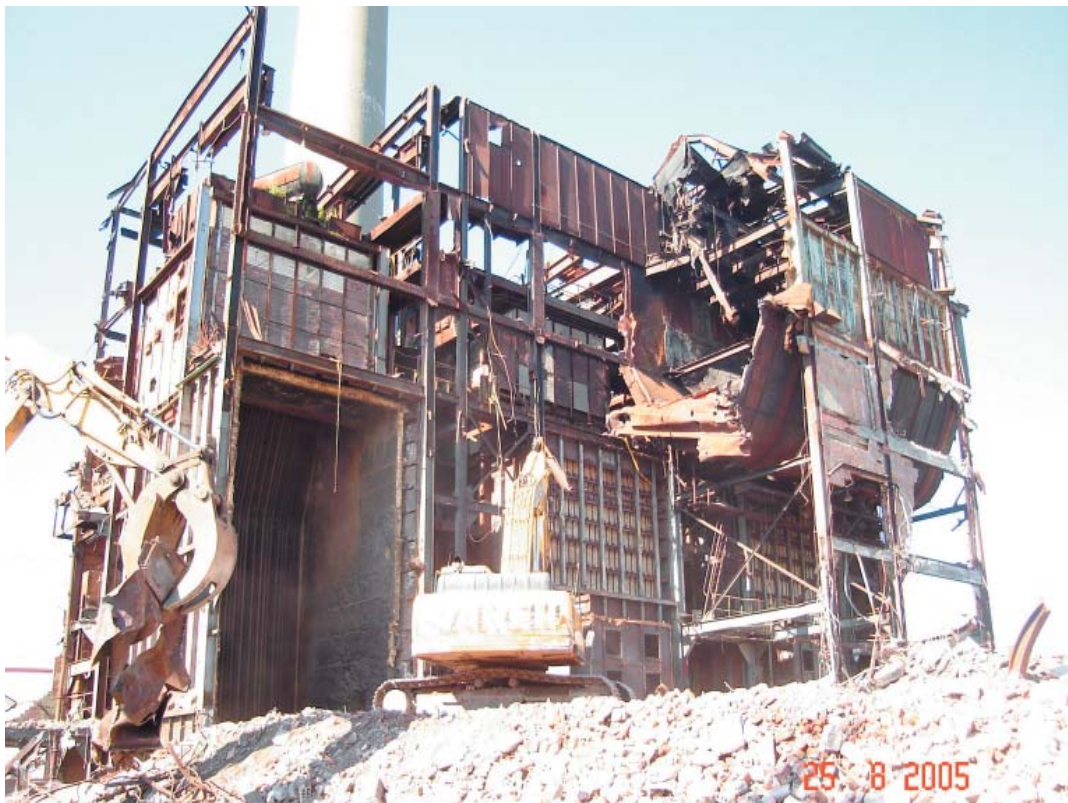
Photo 15 Demolition of south boiler house.
