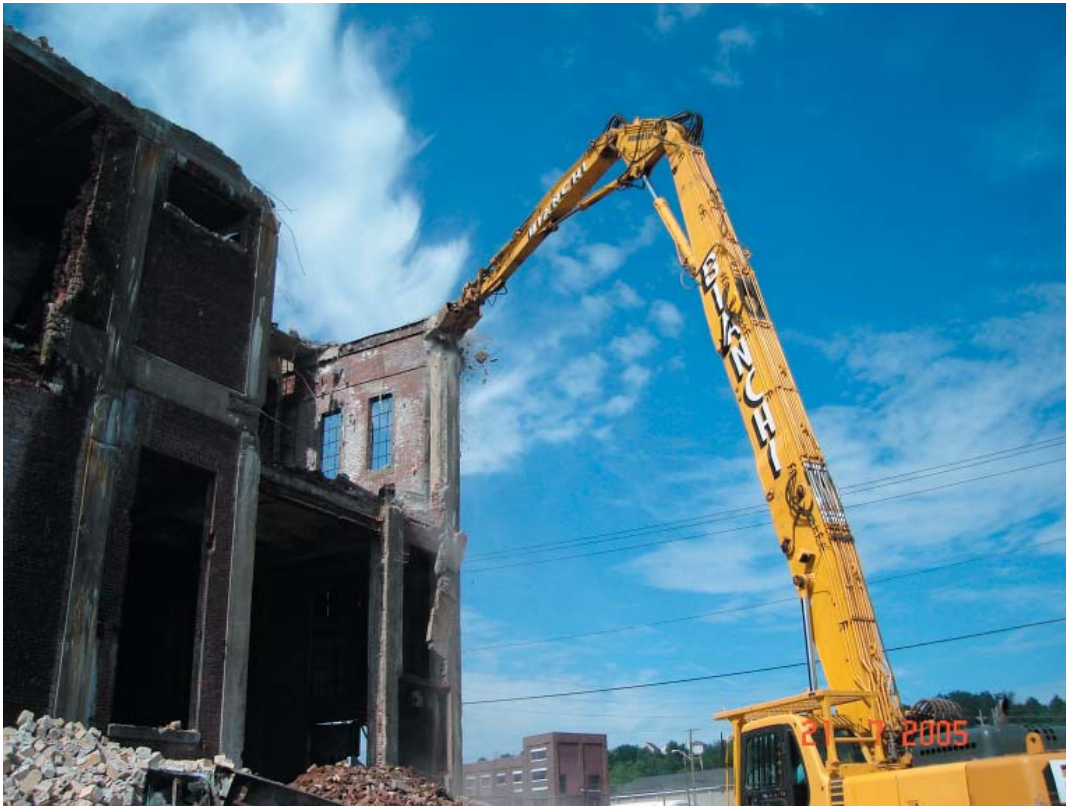
Photo 9 Demolition of north boiler house.
