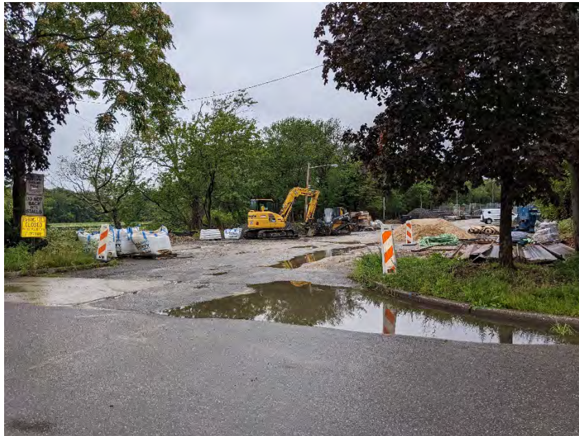
Photograph1: View of the Site, facing northeast.
