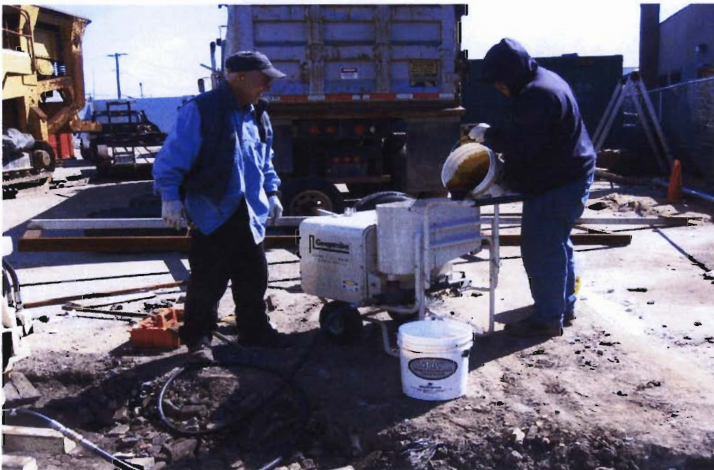
Photograph No. 6 - Injection of Metals Remediation Compound in April/May 2005 at subgrade impacted soil source areas and at southwest property perimeter.
