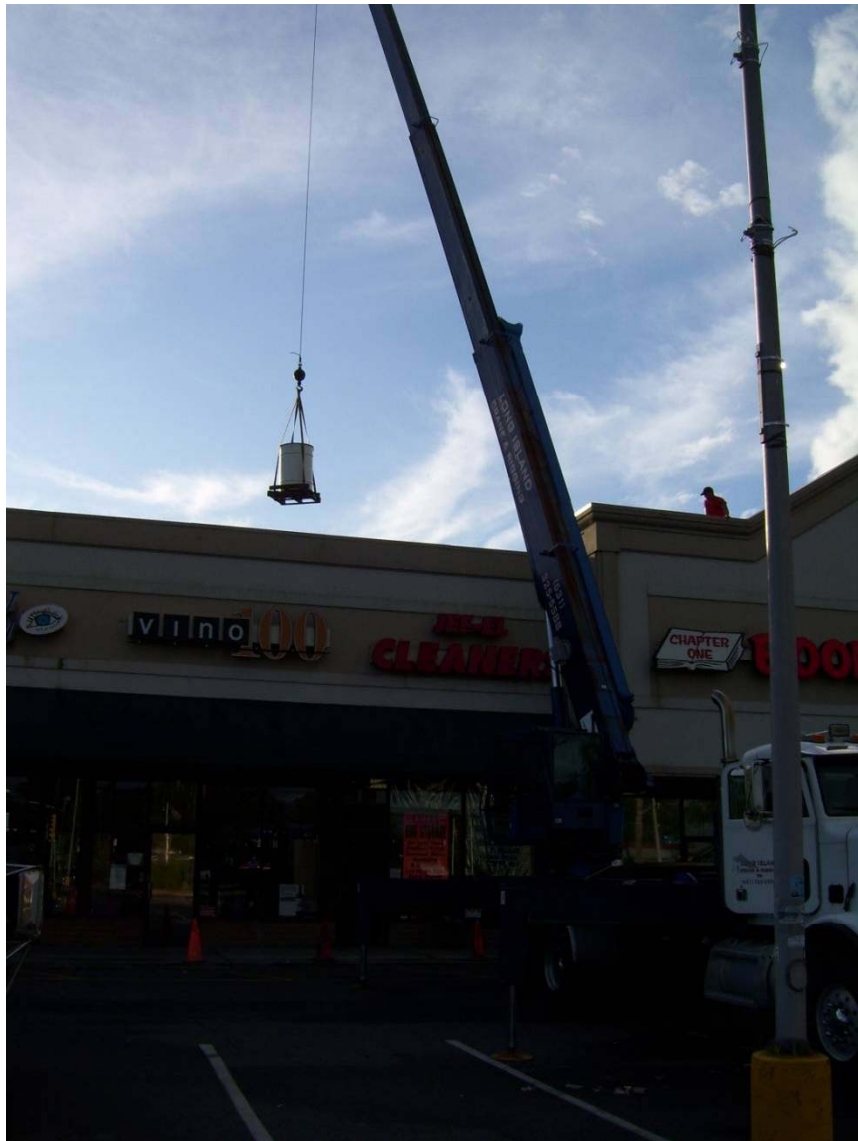
Photograph 3: Vapor-Phase Carbon Drum being hoisted onto the roof.
