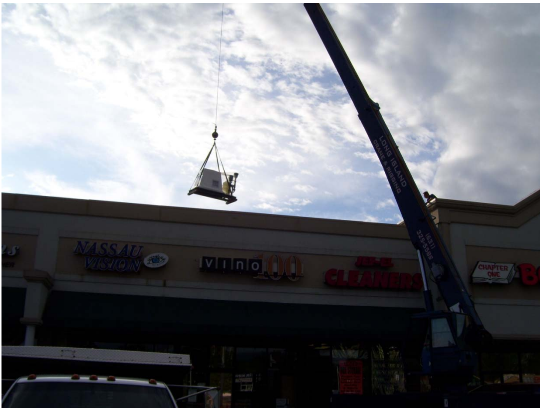
Photograph 2: SVE Blower Package being hoisted onto the roof.
