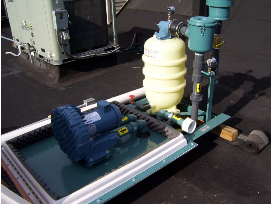
Photograph 4: SVE Blower Package in place on roof, prior to piping being installed.
