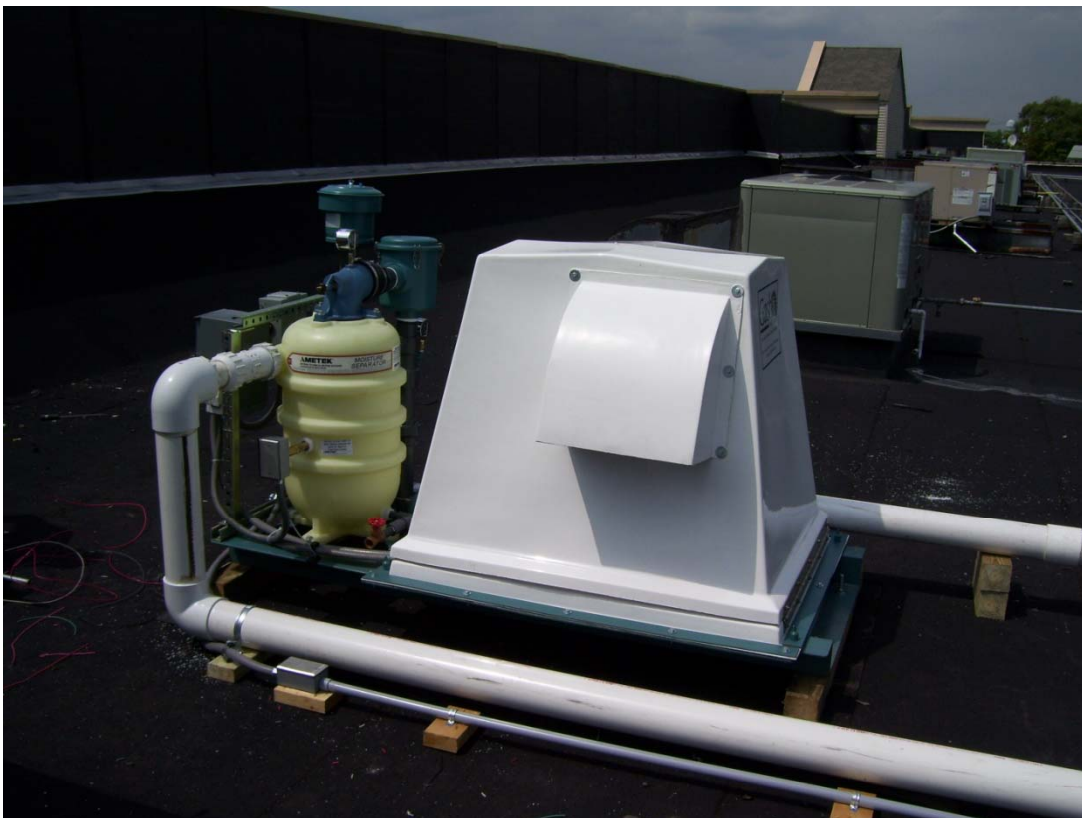
Photograph 5: SVE Blower Package after installation with fiberglass enclosure in place.
