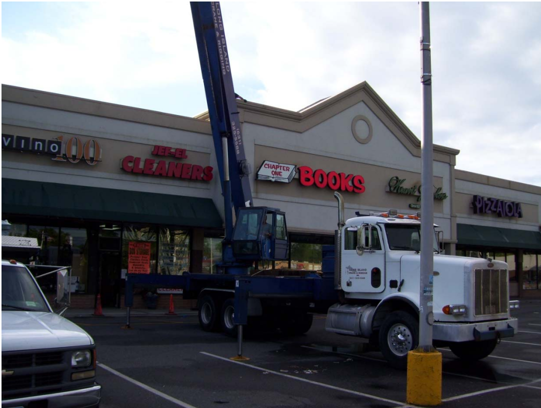
Photograph 1: Crane that was used to hoist equipment onto the roof.
