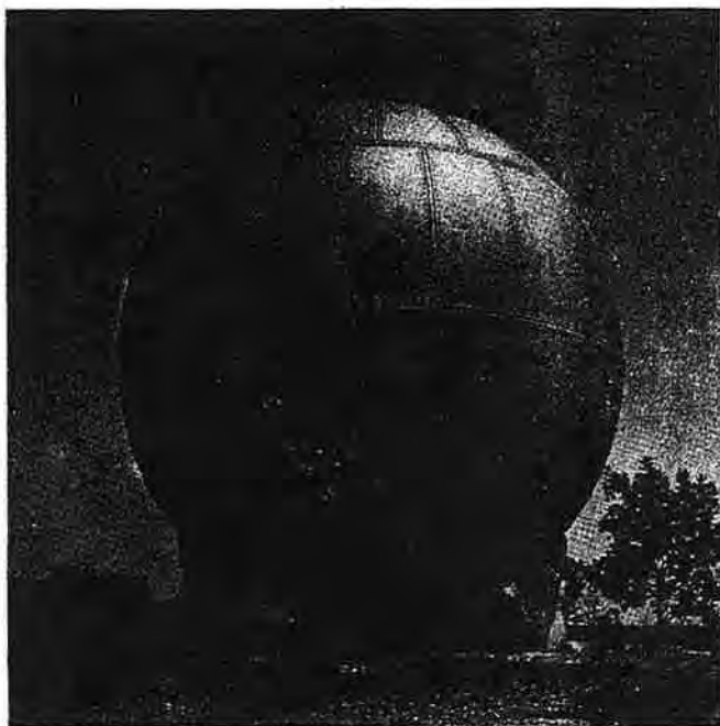
FIG. 27. Hortonsphere High Pressure Gas Holder, 57.5 feet in Diameter. (Courtesy of Chicago Bridge & Iron Works, Chicago, Ill.)
