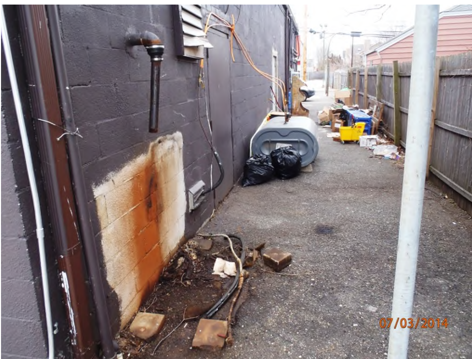
Photograph 2: Alley behind the south Site building. White patch on wall at left denotes the former location of the removed heating oil AST. B4 was installed directly beneath this patch. Photographer facing south.
