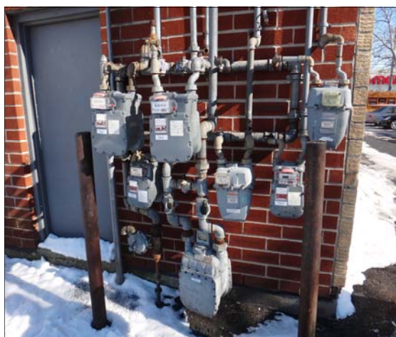
TYPICAL VIEW OF GAS MAIN WITH TENANT METERS FOUND ON SITE
