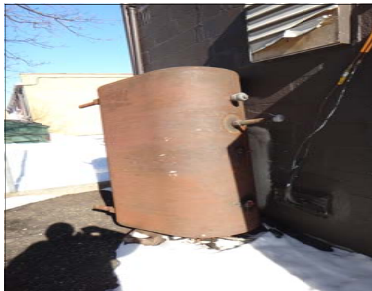
VIEW OF DRY CLEANERS OIL FIRED STEAM BOILER
