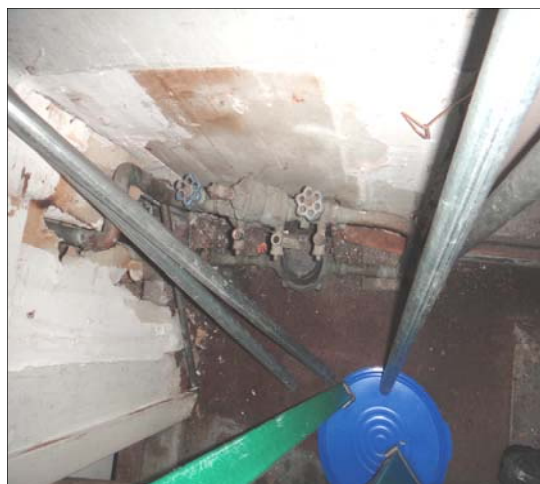
TYPICAL VIEW OF COPPER WATER MAIN AND METER ON SITE
