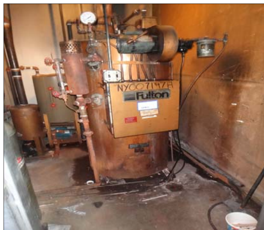
VIEW OF DRY CLEANERS OIL FIRED STEAM BOILER
