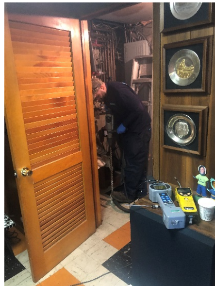
Photo #8: Sub-slab sample probe installation at 5 University Place
