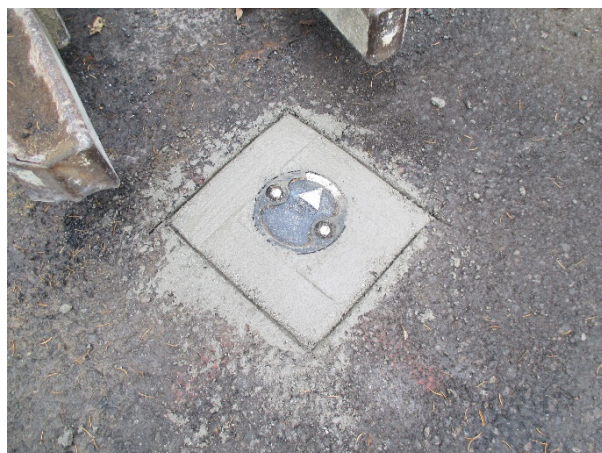
Photo #10 (11/12/2020): Completed monitoring well (typical)
