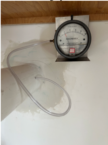
SSD-1 Pressure gauge (Dwyer Magnehelic)
