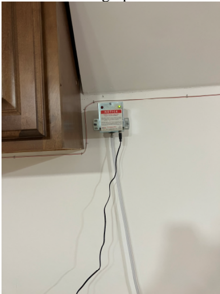
System Radon Alarm
