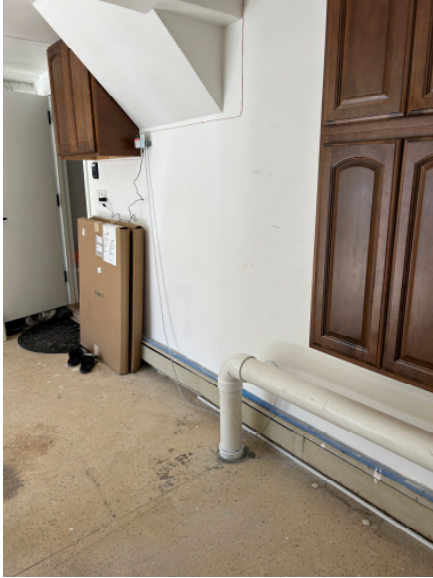
Interior SSD-1 system configuration in garage.
