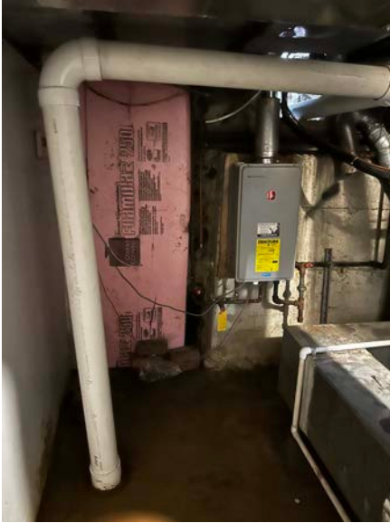
Interior SSD system configuration and penetration through wall.
