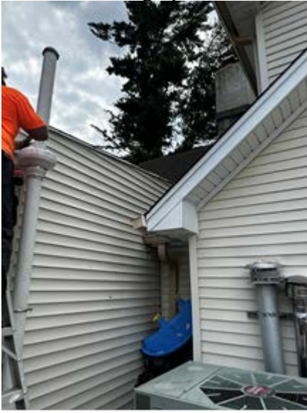
View of SSD-1 vent pipe above the roof
