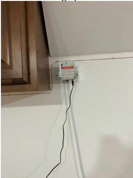
System Radon Alarm
