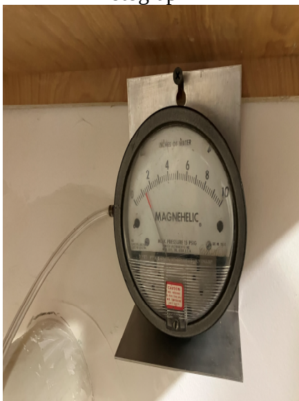
SSD-1 Pressure gauge (Dwyer Magnehelic)
