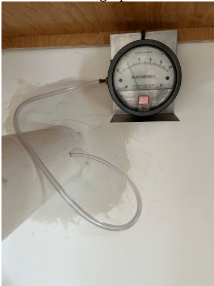
SSD-1 Pressure gauge (Dwyer Magnehelic)
