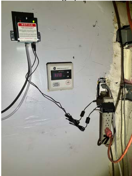
System Radon Alarm
