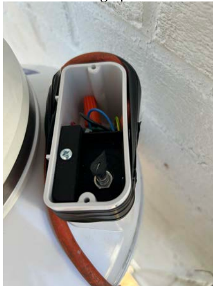
Inside configuration of exhaust fan Radon Away model GP501c.
