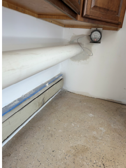
View of the PVC pipe penetration exiting the east wall of the house and the pressure gauge.
