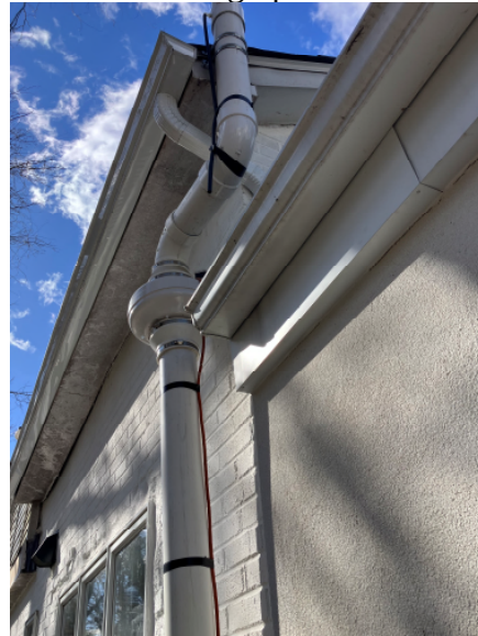
View of SSD-1, exhaust fan, including vent pipe above the roof.
