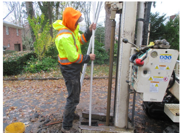
Photo #8 (11/12/2020): Off-site monitoring well installation on University Place (typical).
