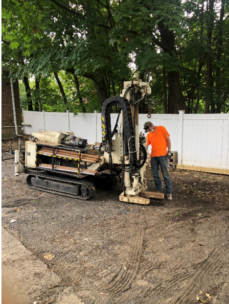
Photo #1 (8/31/2020): Soil boring via direct-push drilling (typical)
