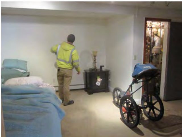
1. Performance of a Ground Penetrating Radar (GPR) survey to select safe location for sub slab drilling.
