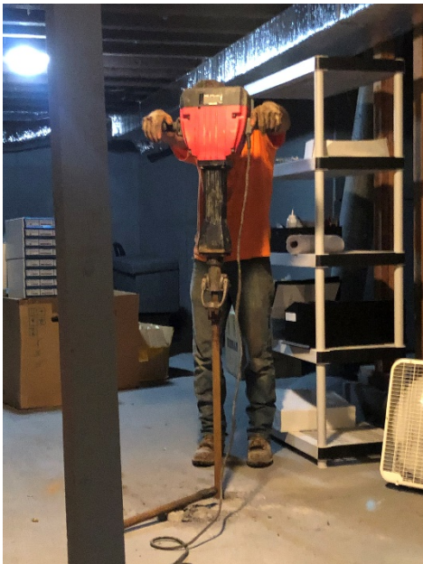
Photo #3 (9/1/2020): Soil boring inside building
