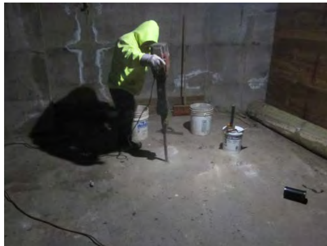
2. View of drilling equipment into a building slab.
