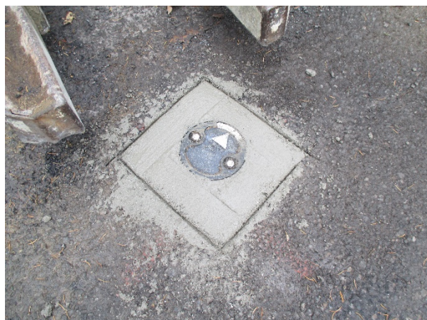
Photo #10 (11/12/2020): Completed monitoring well (typical)
