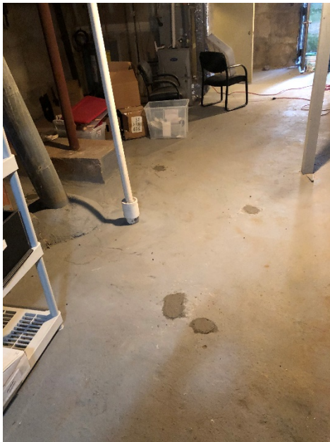
Photo #5 (9/3/2020): Patched boring location inside building
