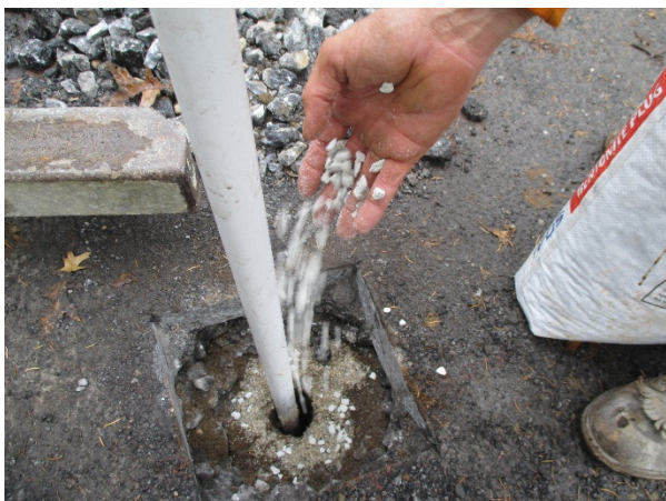
Photo #9 (11/12/2020): Installation of bentonite seal during monitoring well installation (typical)
