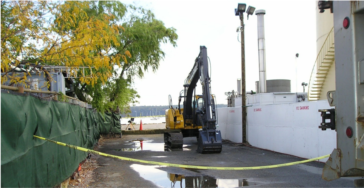
Photograph No. 1 Area to be excavated, facing east
