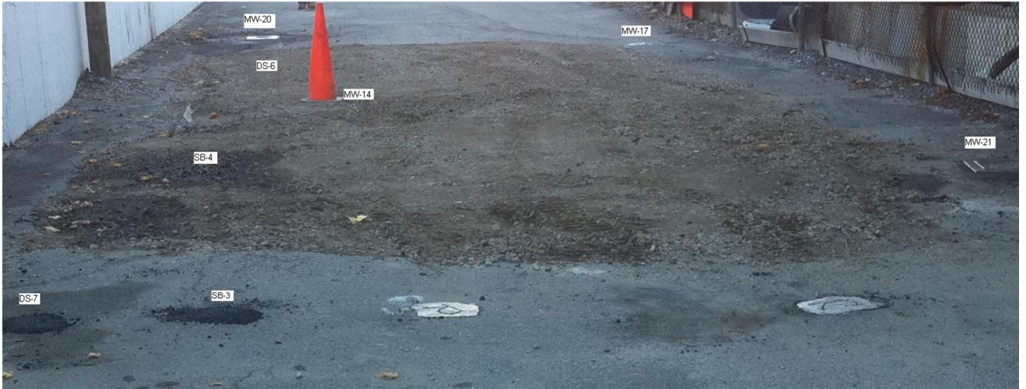
Photograph No. 5 Discrete Sampling and soil boring locations, facing west
