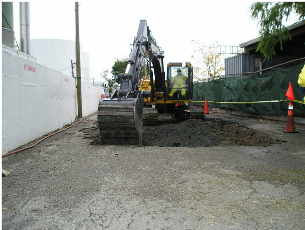
Photograph No. 2 Beginning of excavation - breakout of asphalt facing west
