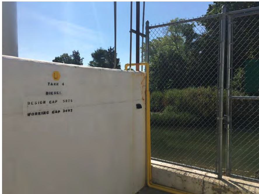
Figure 6: View of secondary containment wall for eastern AST area along southern property boundary.
