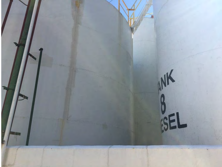
Figure 7: Image of ASTs on eastern portion of the property.
