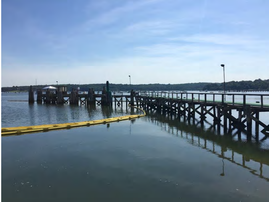
Figure 25: View of dock to the east of the subject site with spill containment booms in place.
