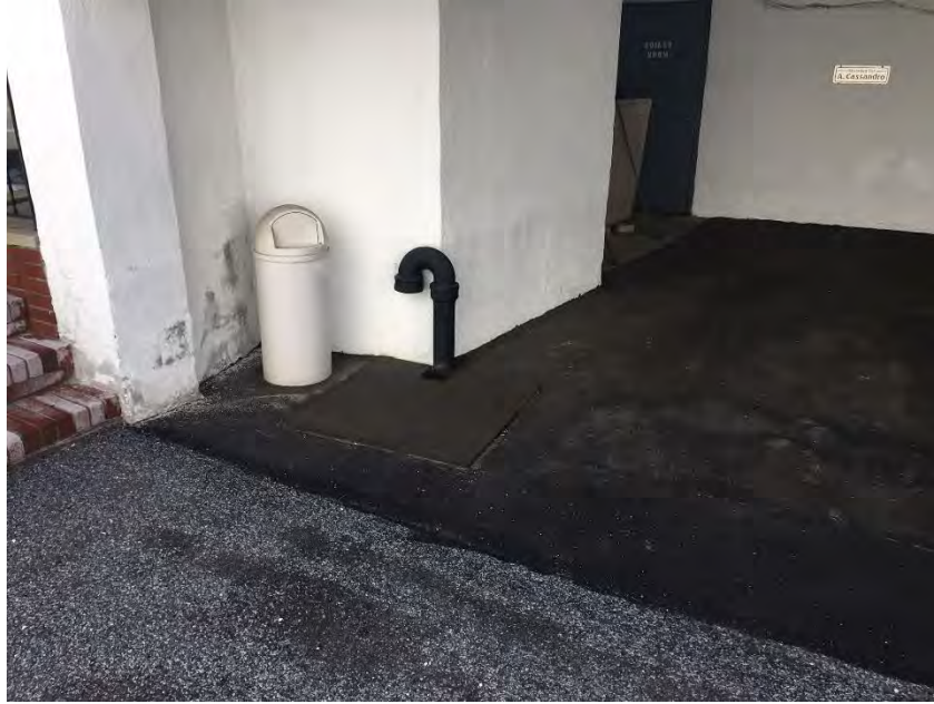
Figure 1: Vent pipe for sewer adjacent to office building.
