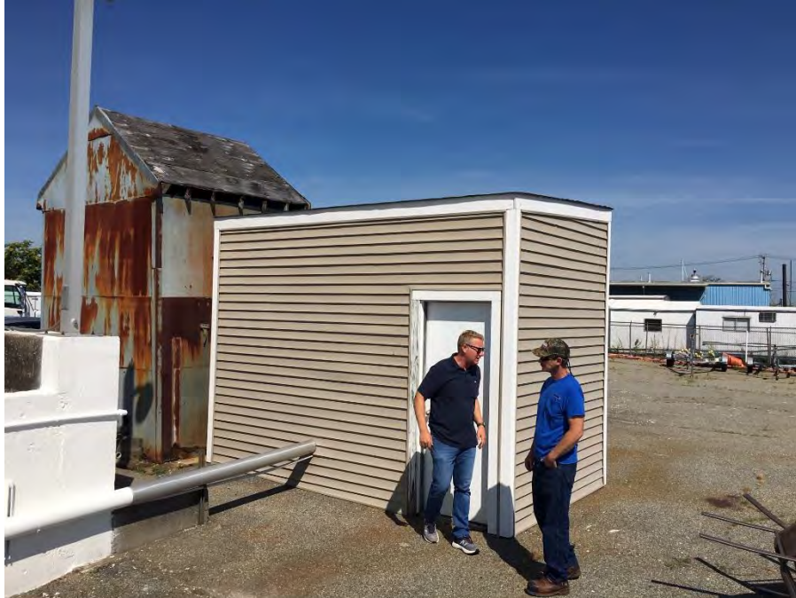
Figure 27: Water treatment system shed.
