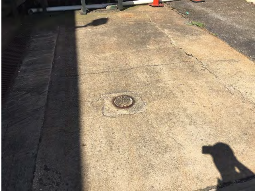
Figure 13: Image of monitoring well near central portion of the property.
