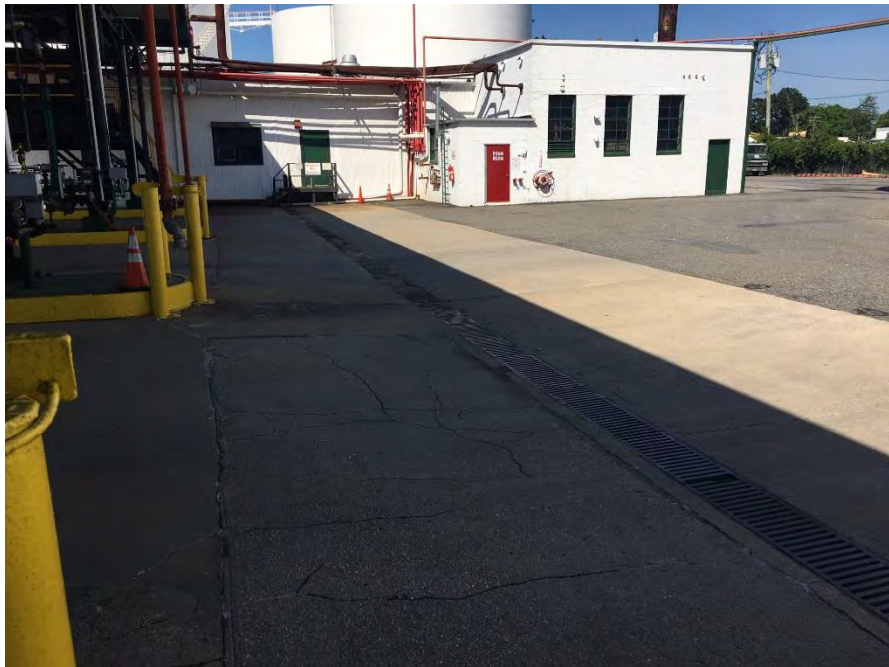
Figure 10: Trench drain located in central portion of the site.
