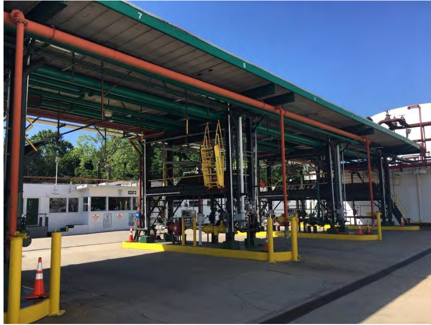
Figure 11: Delivery truck filling area.
