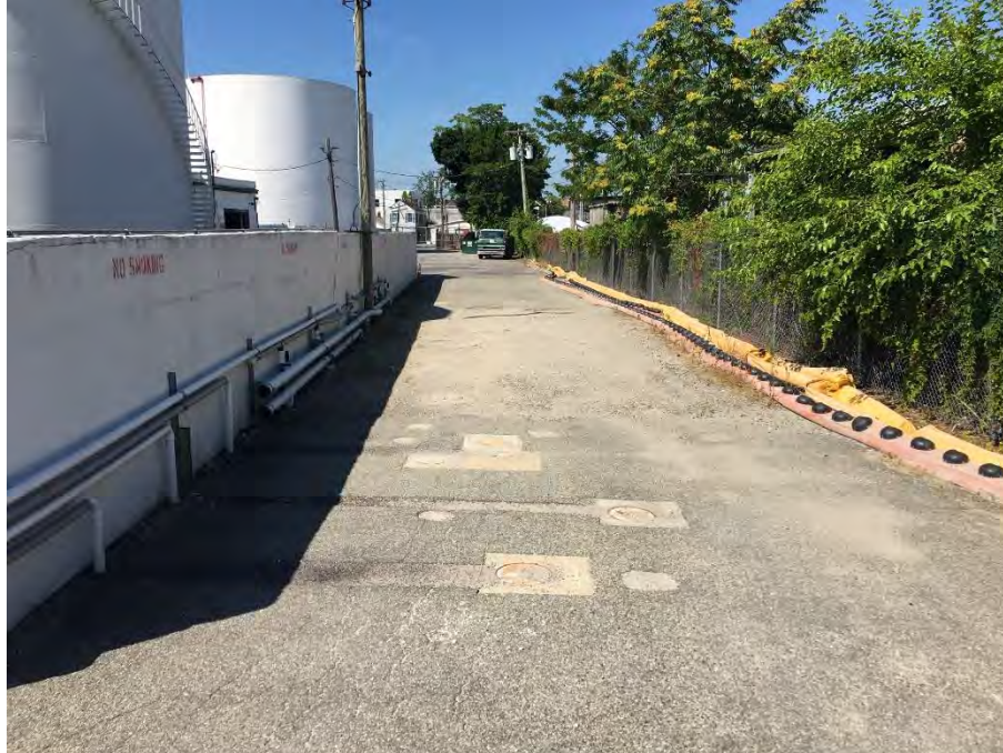
Figure 31: Network of monitoring wells in location of chlorinated solvent spill.
