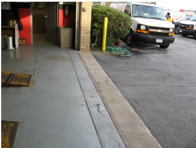
Photo 1: Trench drain filled with concrete within the vehicle maintenance garage.
