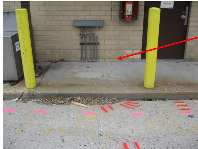
Photo 5: View of the south side of the building showing the five electric conduits and two cut UST vent lines.
