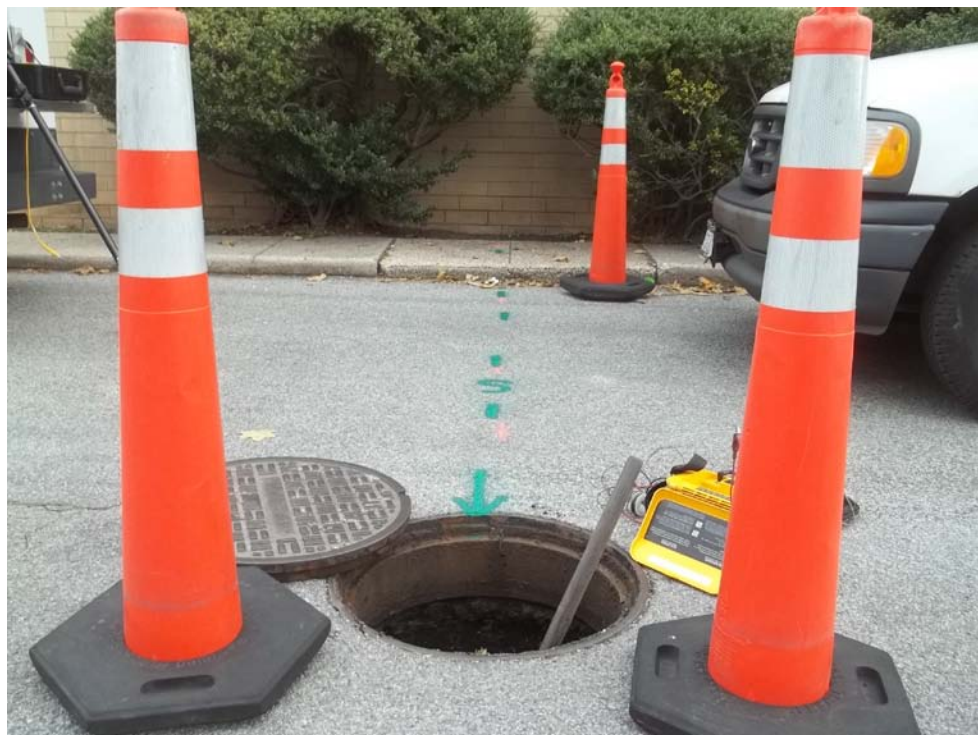
Photograph 4: Drywell piped to area of former oil-water separator/drainage system in maintenance bay.
