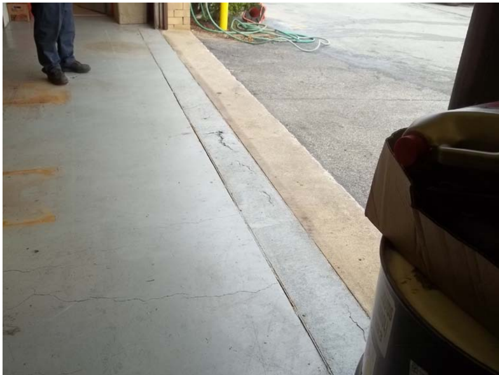
Photograph 2: Location of former trench drain in maintenance bay.
