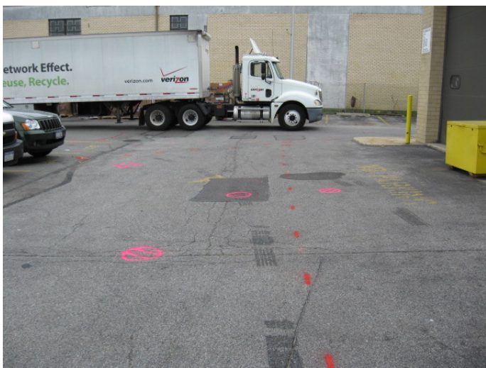
Photo 3: View looking south. The asphalt patch in the center of the photo represents the former location of the 280-gallon waste oil UST. The electric line servicing the light pole located opposite the tractor trailer is visible immediately west of the asphalt patch.
