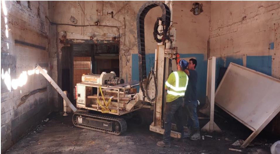
31. Location of SB-5 in southwest area of building facing south
