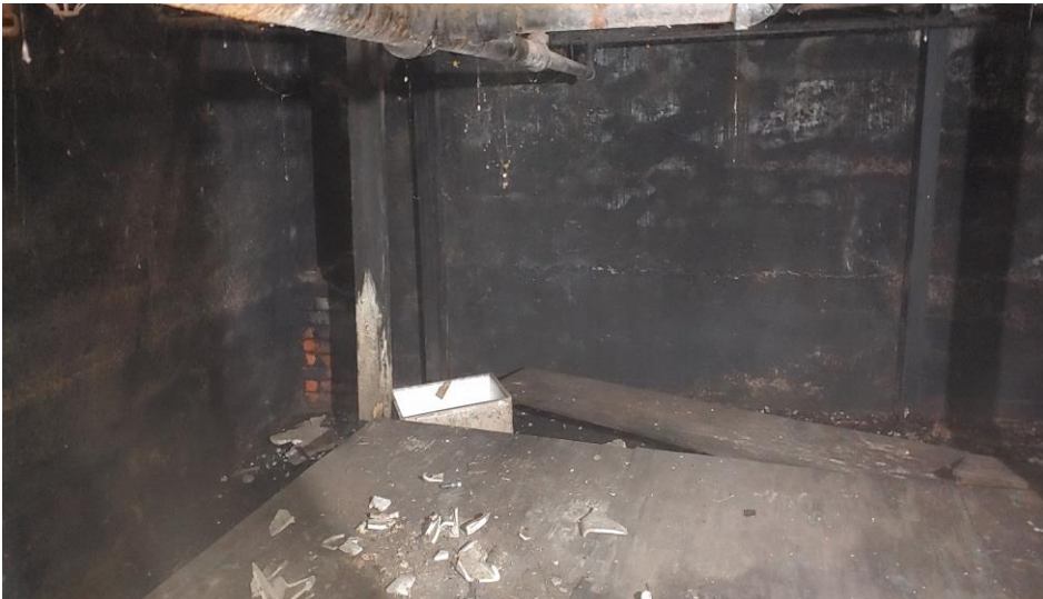
3. View of wood covering sump in basement
