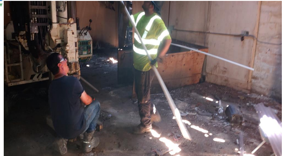
24. Installation of temporary well in SB-3
