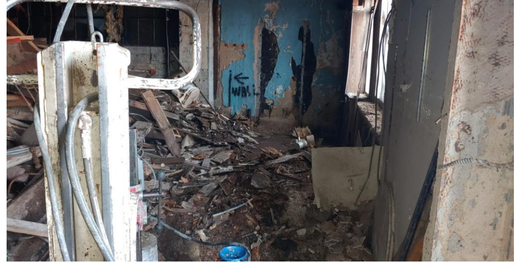
14. View of soil boring SB-1 in northeast corner of building
