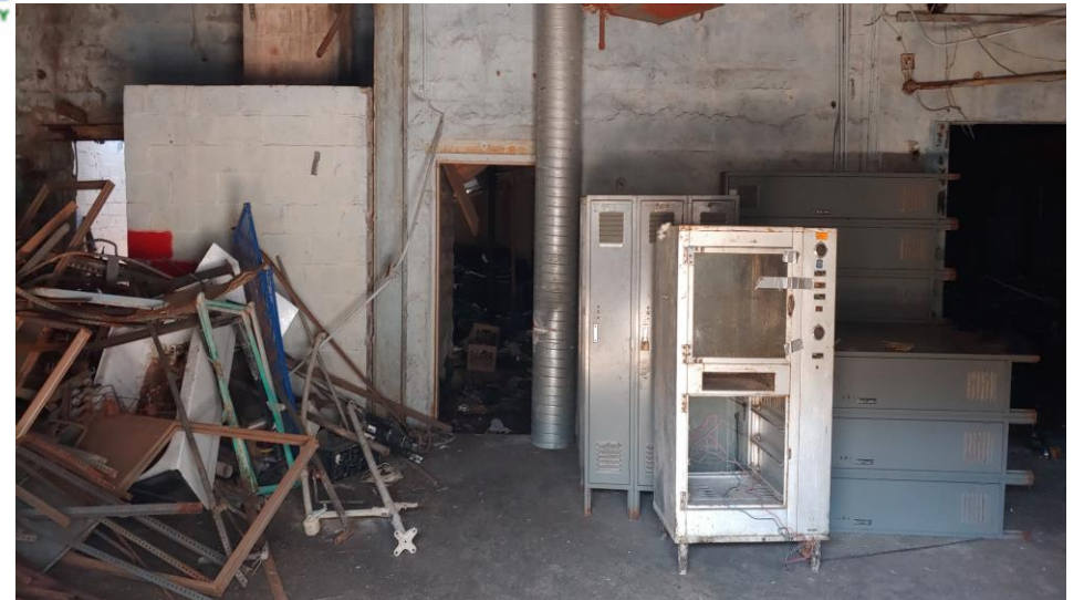
12. South-West middle of building
