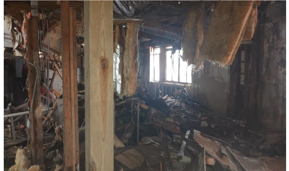
6. View of northeast (front) area inside the building
