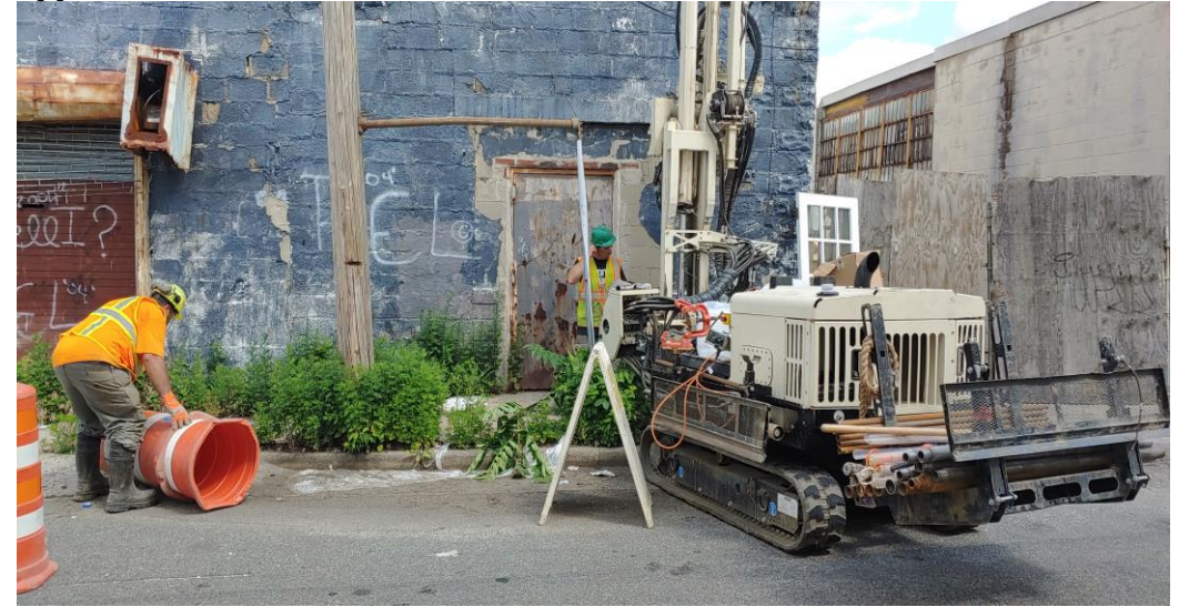
14. Location of Borehole BH-4 from south facing north
