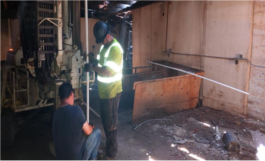
25. Installation of temporary well in SB-3
