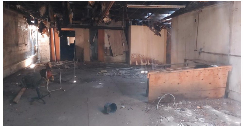
8. View of east-middle of building; note entrance to basement
