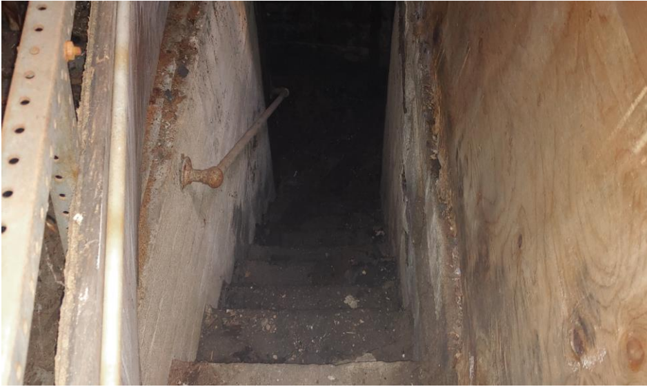
1. Stairs to small basement center of building
