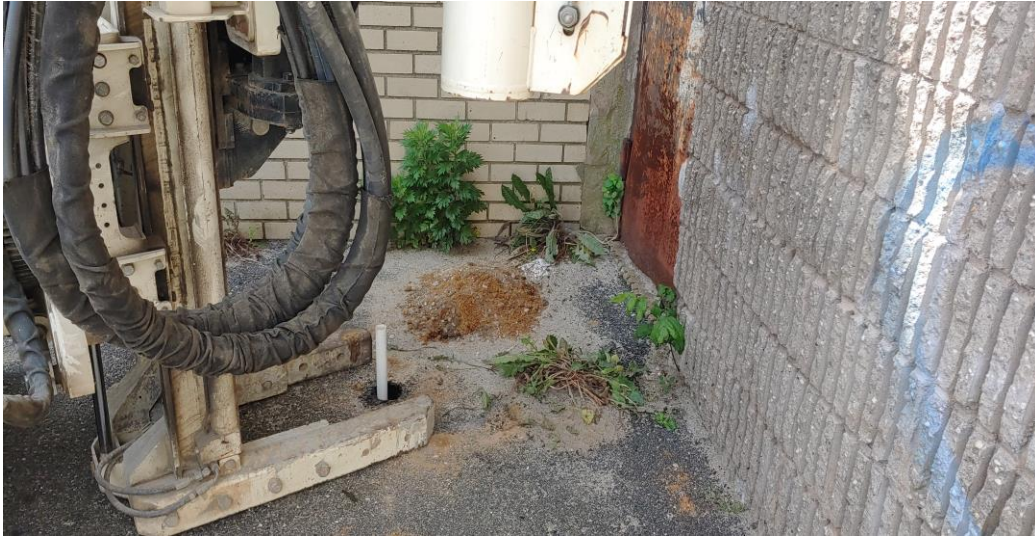
13. Temporary well installed in BH-3
