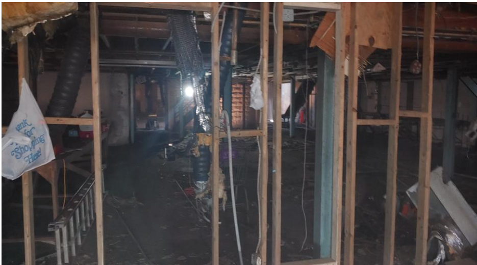
7. View inside building from northeast front corner facing south towards the middle of the building
