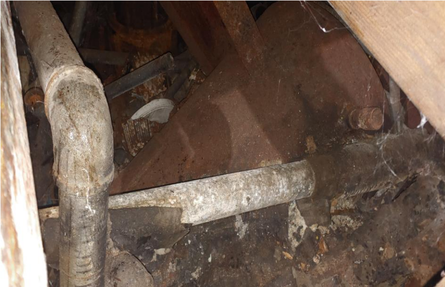
5. Piping and possible drum/tank in sump in basement
