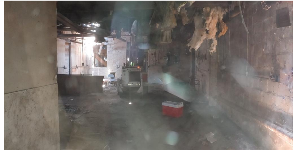
20. Location of Soil Boring SB-3 in the middle east side of building adjacent to the basement
