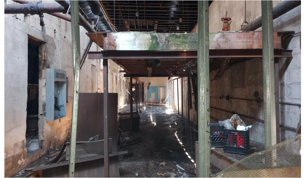
10. Middle of building
