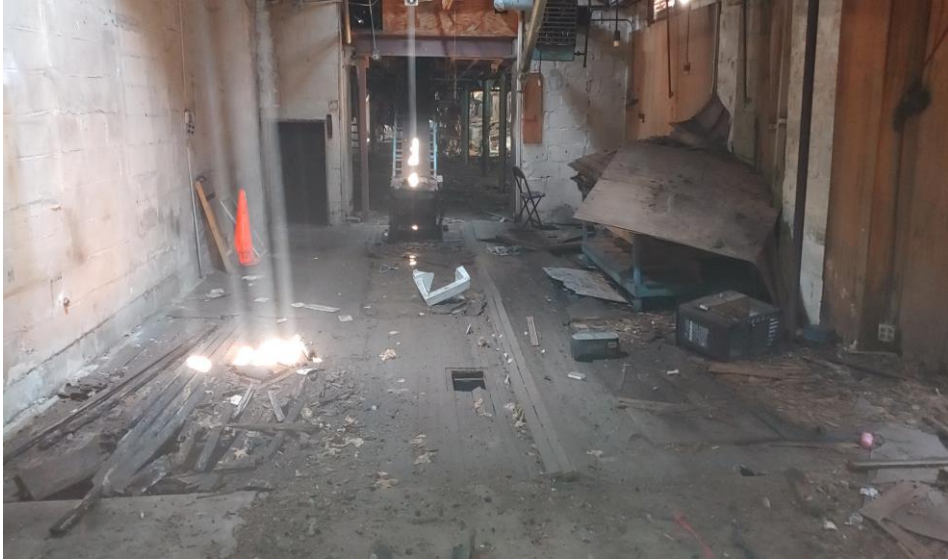
9. Middle of building
