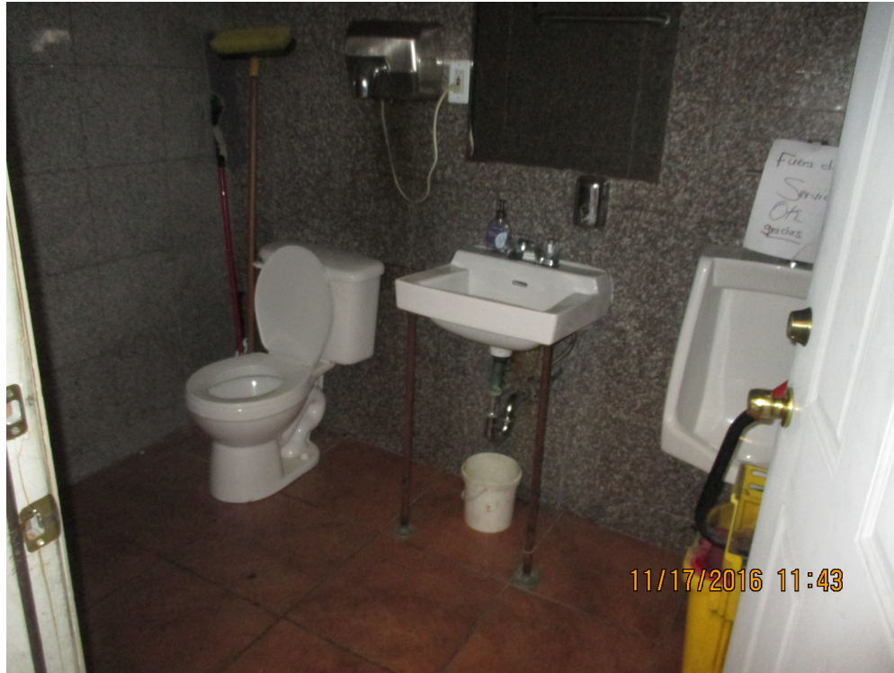
Typical toilet with newer finishes.
