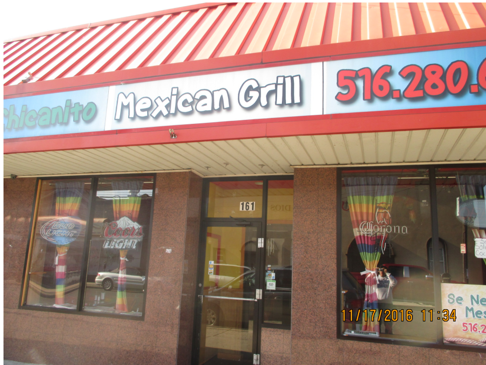
Storefronts have anodized aluminum windows and doors with rubber gaskets.
