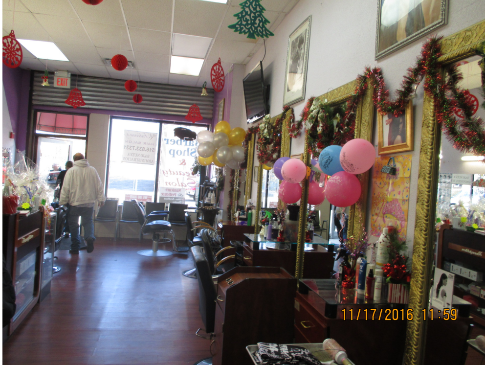
Finishes in Commercial Retail Building – flooring on concrete with sheetrock walls and ceiling tile – all non-asbestos – typical for all spaces
