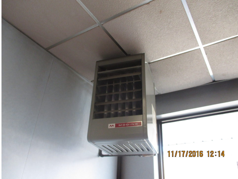
No ACM associated with unit heaters.
