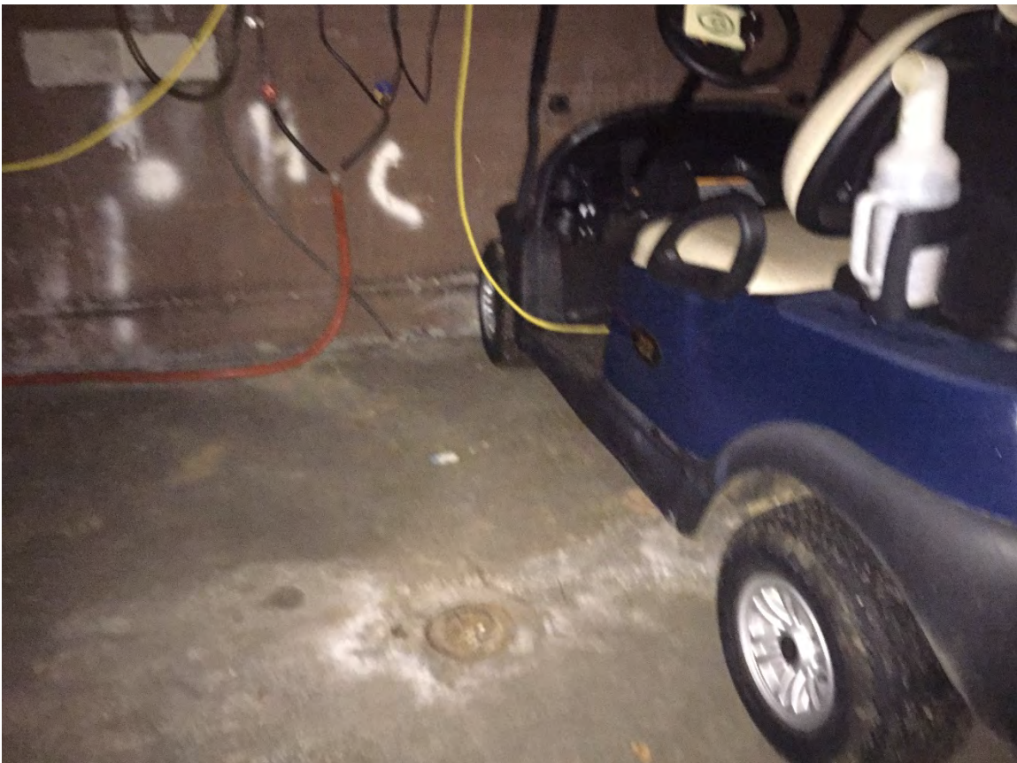
Photograph No. 12: Typical interior small diameter floor drain in the golf cart garage.
