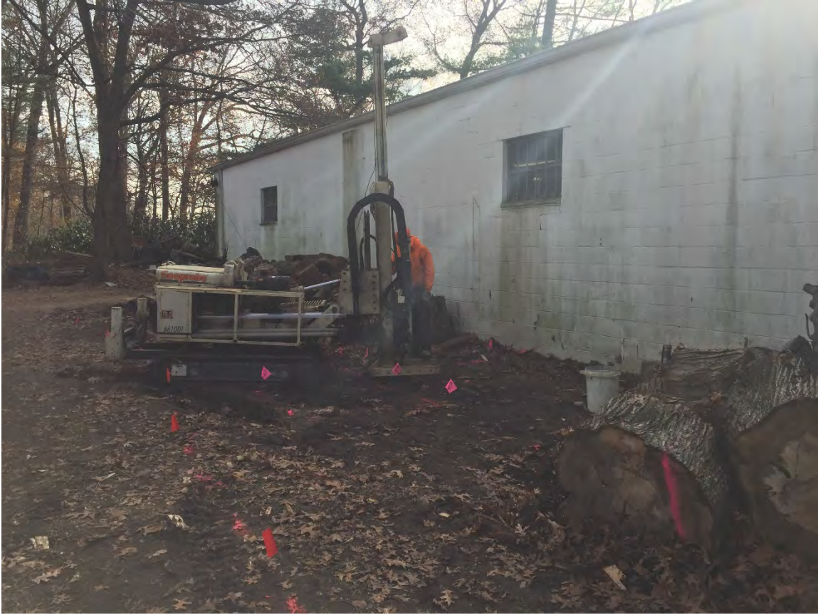
Photograph No. 5: The installation of soil borings proximate the 550-gallon fuel oil UST.
