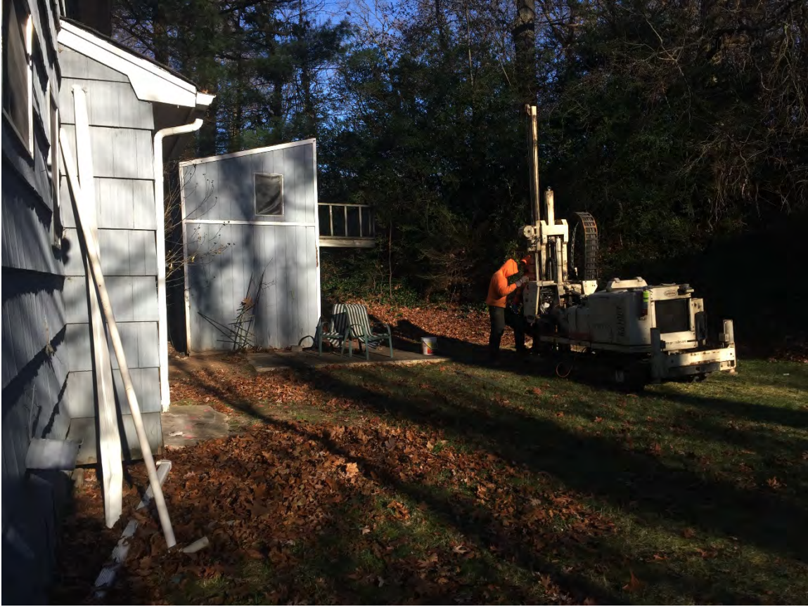
Photograph No. 9: Insulation of a soil boring in the rear yard of the stand alone dwelling.
