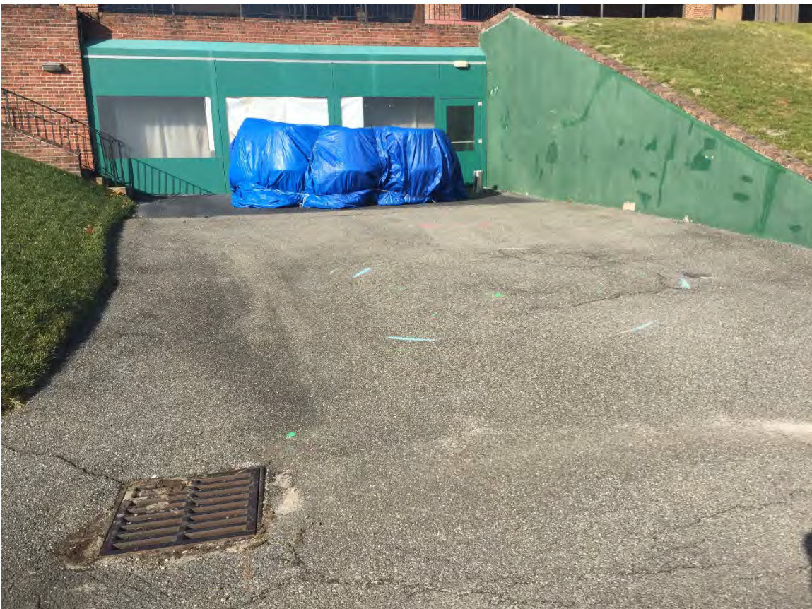
Photograph No. 14: The location of an at-grade drywell and its interconnected overflow.
