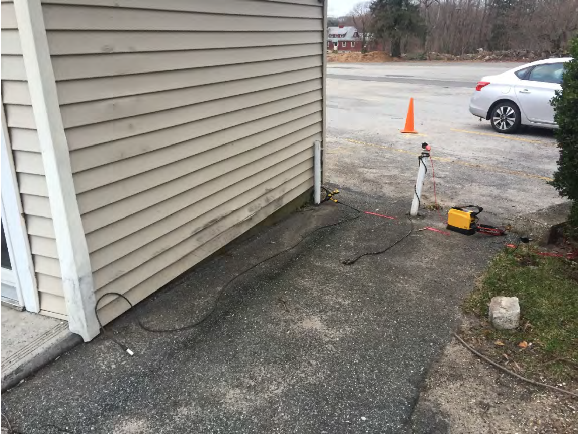
Photograph No. 3: Typical suspect piping investigated during the geophysical survey.
