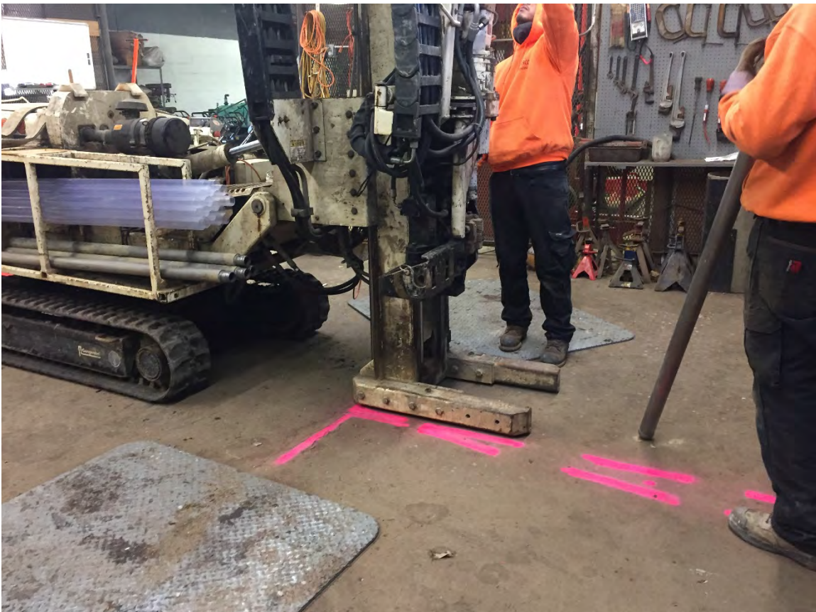
Photograph No. 6: The installation of soil borings proximate the hydraulic piston lifts.
