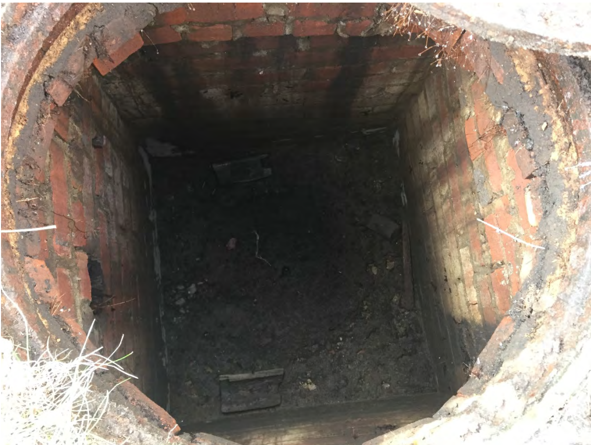
Photograph No. 16: The interior of the catch basin along the driveway and a pipe within.
