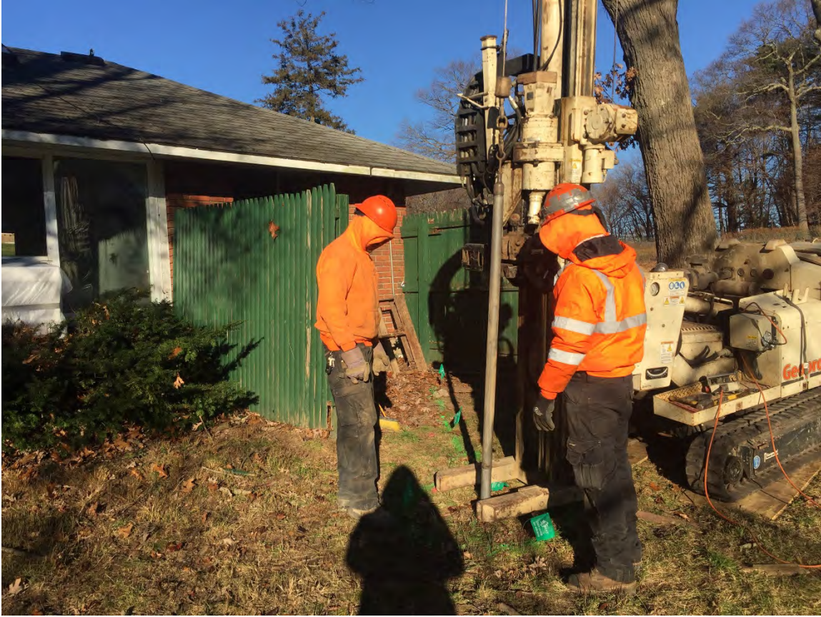
Photograph No. 7: Installation of a soil boring through the cover of a sanitary structure.
