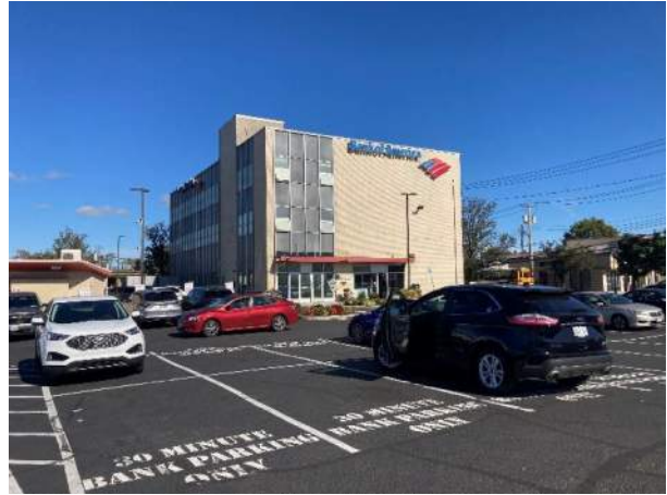
Photo 14. Looking at the adjacent property located to the north.
