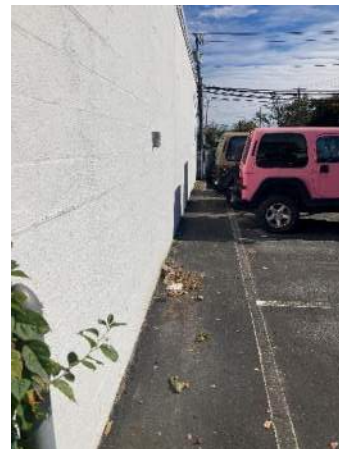
Photo 4. View looking toward the east along the south side of the building. The building is the end of the property line.
