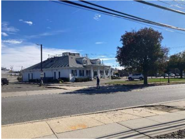
Photo 13. View of the property to the east, across Jerusalem Avenue.
