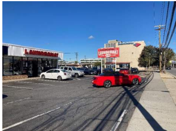
Photo 10. Front parking area along Jerusalem Avenue.
