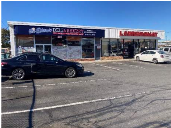
Photo 1. View of the 1-story building on the Site.
