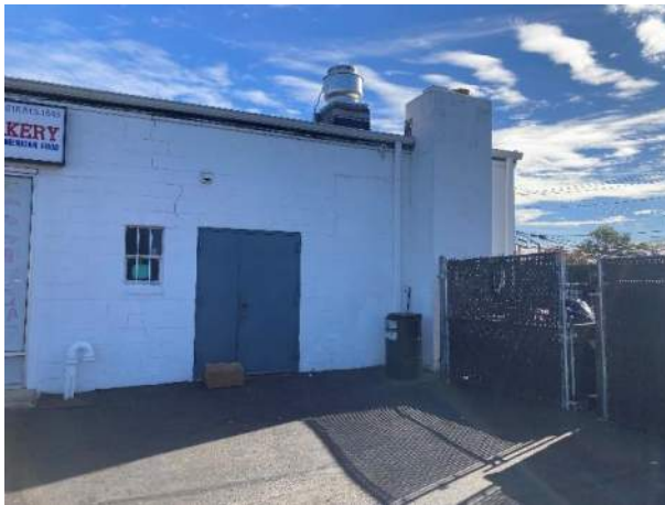
Photo 9. Chimney that is no longer being used. Behind this area of the building is the kitchen for the deli.
