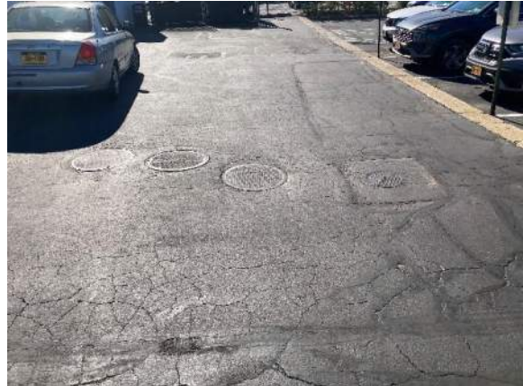
Photo 8. Sewer connection cleanout in rear parking area.
