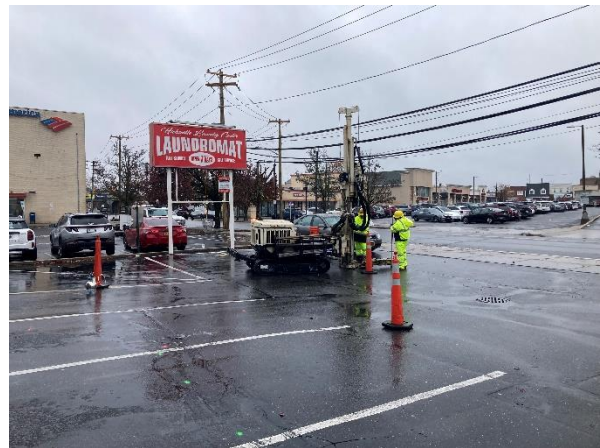
Photo 2. Installing soil boring SB-2.
