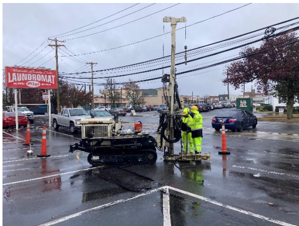
Photo 5. Installing the temporary groundwater monitoring well GW-1.
