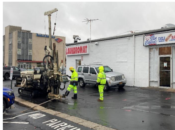
Photo 6. Preparing to install soil vapor point SV-3.
