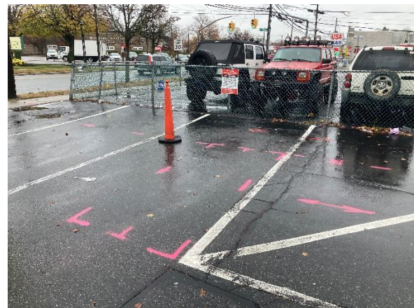
Photo 4. View of the outline of the UST anomaly in the front parking area.
