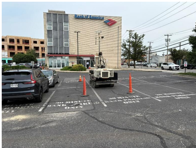
5. View of SI-SB-1 location.
