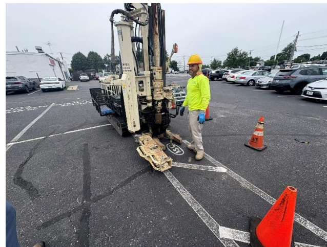
12. View of SI-SB-4 location.
