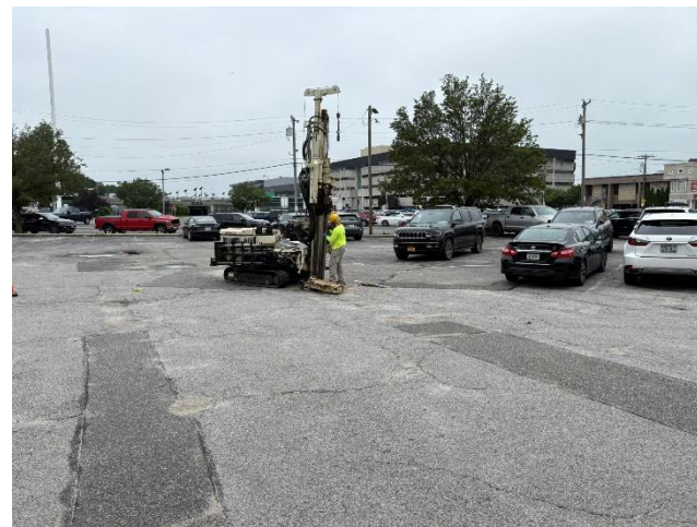
16. View of SI-SB-7 location.
