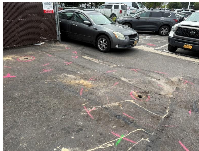
10. View of DW-1 and DW-2 locations.
