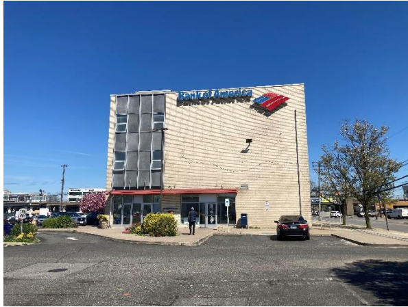
Photo No. 1 – Looking north at the building from the south side of the Site.
