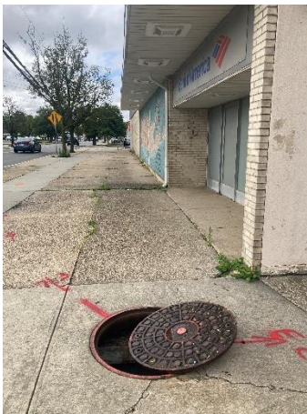
Photo No. 5 – View of a manhole cover not associated with a drain.
