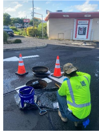
Photo No. 2 – Working around SS-1 associated with the on-site septic tank.
