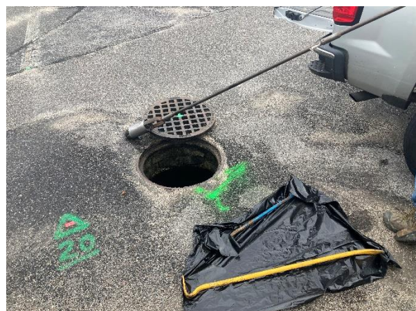
Photo No. 6 – View of SW-1 on the southern end of the Site.
