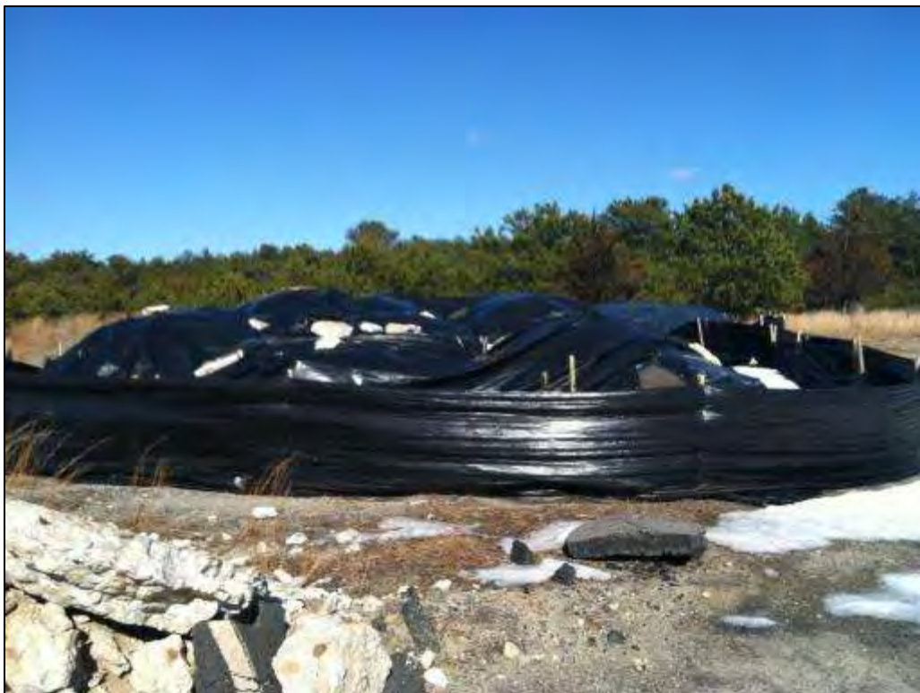
Photo 14 – Soil stockpile covered with polyethylene sheeting and surrounded with silt fence.
