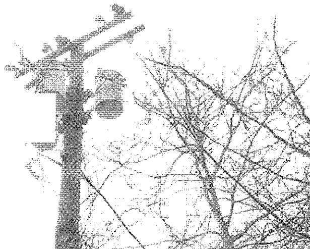
7. POLE-MOUNTED ELECTRICAL TRANSFORMERS LOCATED AT THE SITE.
