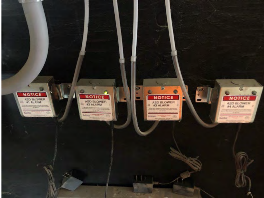
Photograph 1: View of the alarms for the SSDS fans. Only the alarm for SP2 is plugged in since this is the only required SSDS fan to be operating.
