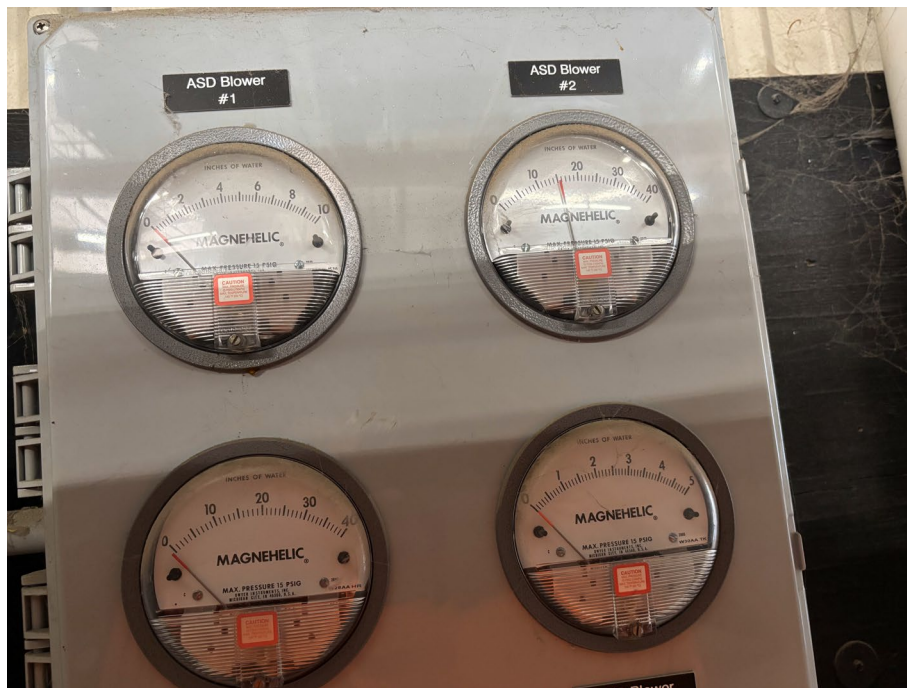
Photograph 1: View of the vacuum gauges for the SSDS fans. Only SP2 is showing vacuum.
