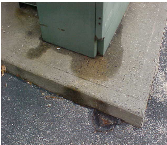
Pad-Mounted Transformer – Slight Staining
