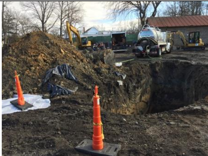
PHOTO 5: Stockpiled soils associated with UST removal. UST pump-out being completed in background to remove sludges and UST contents.
