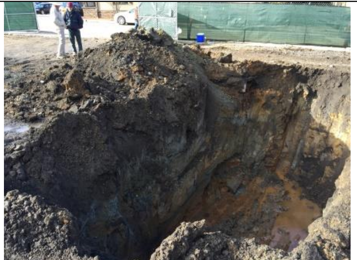
PHOTO 6: View of the final excavation following removal of UST and associated impacted-soils.
