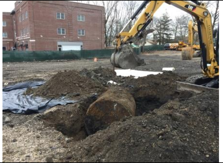
PHOTO 2: Begin removal of the single-walled 550-gallon UST utilizing excavator.
