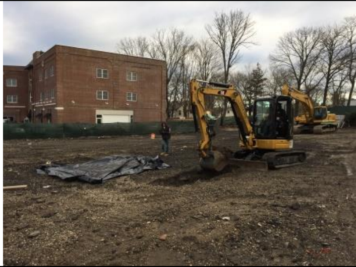
PHOTO 1: Begin excavation at the geophysical survey confirmed Underground Storage Tank (UST) location.
