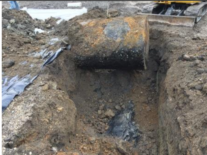
PHOTO 3: Removal of the 550-gallon UST and UST grave; note lack of heavily stained soils/saturated soils
