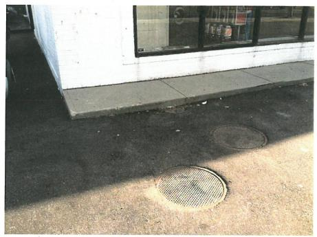
Photo 7 – Suspected septic tank to the north of the laundromat
