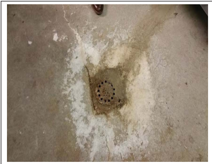
FLOOR DRAIN IN BASEMENT
