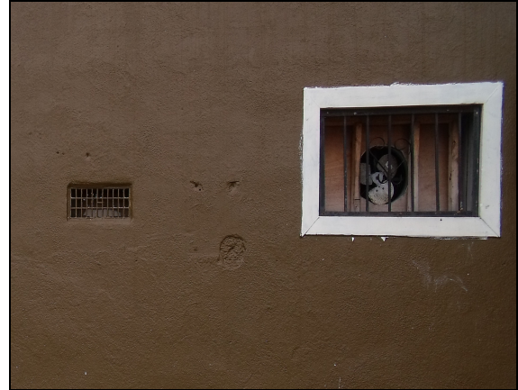
Photo #2: Restaurant wall exhaust fan.
