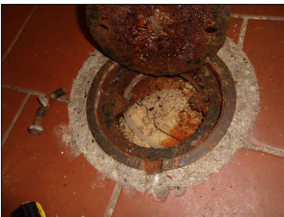
Photo #5: Restaurant basement floor test port.
