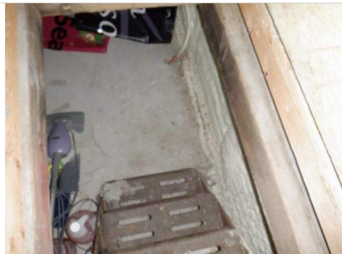
15. Crawl space access
