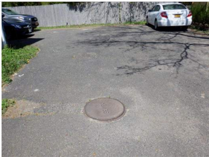
7. Septic cover in driveway
