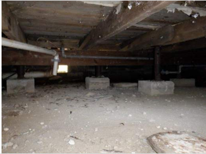
17. Apartment building crawl space
